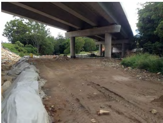
Plate 4.1 UWC construction area through Zones 9 and 10 view to the north
