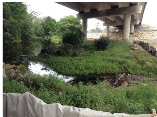
Plate 4.2 UWC construction area through Zones 9 and 10 view to the south
