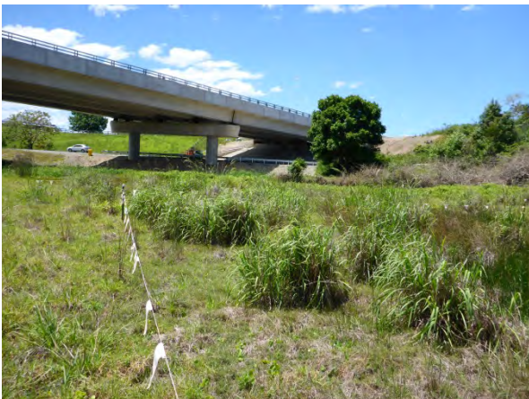
Plate 1.35 Photo point 9 – facing north (December 2017)
