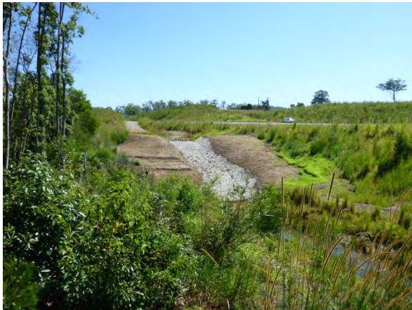
Plate 1.15 Photo point 4 – facing north (December 2017)
