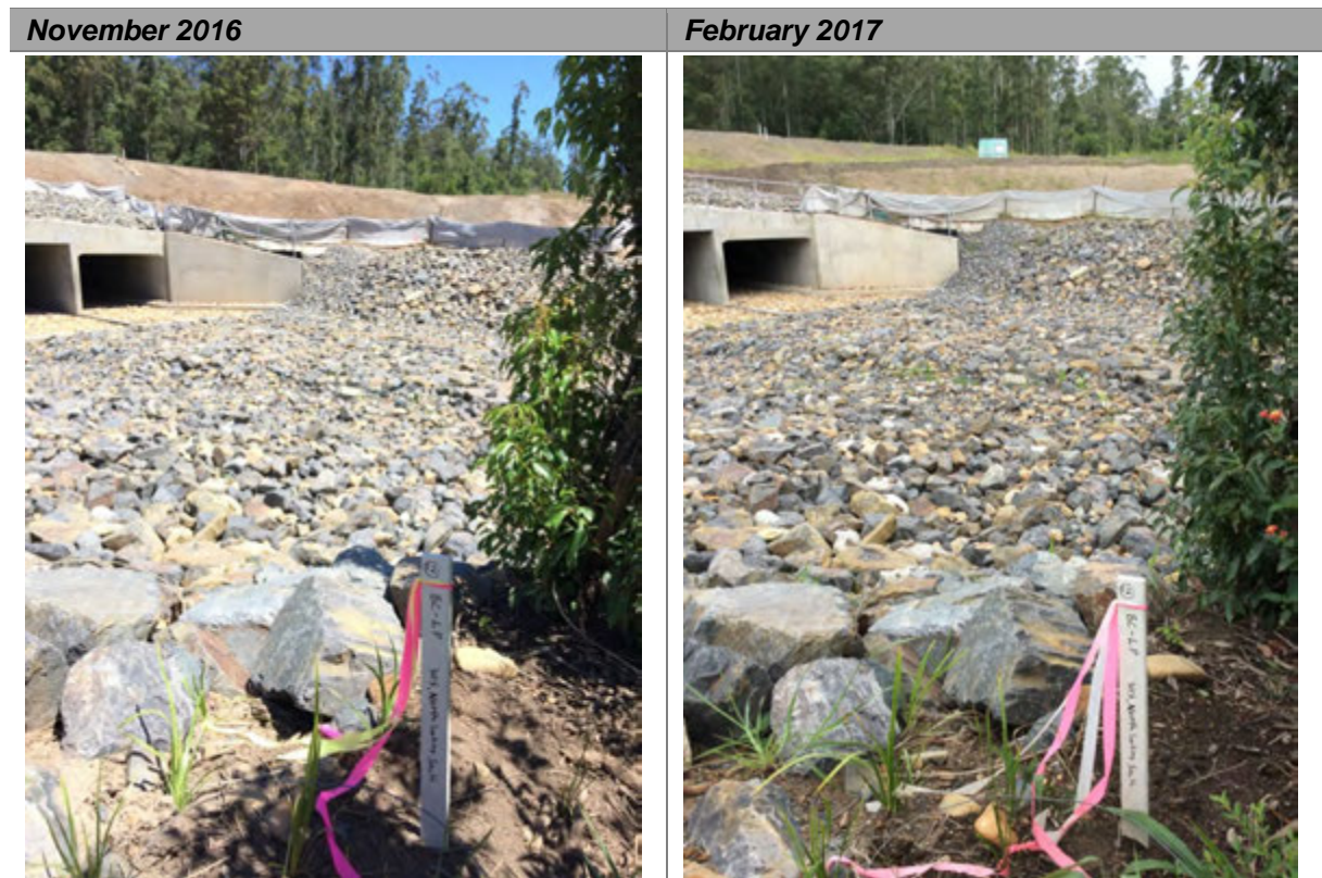
Plate 3.23 Site 12 view to south (Nov 2016)
