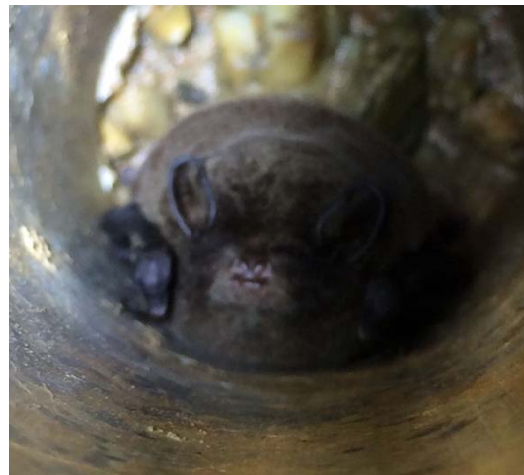
Plate 1.4 Culvert 599222 - Donnellyville. M. australis present in scuppers.
