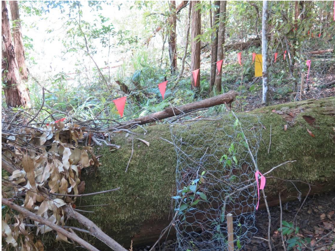
Plate 11: Receival Site 3. Exposed to the east by highway alignment, in background. A buffer of forest ~15m wide separates receival area from construction. Feb/2016
