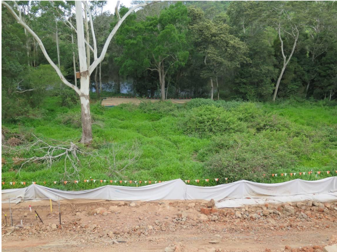
Plate 22: Receival Site 9. Floyds Grass translocation area in background, see light brown shade cloth, about 10 metres from Warrell Creek. Highway in foreground.
