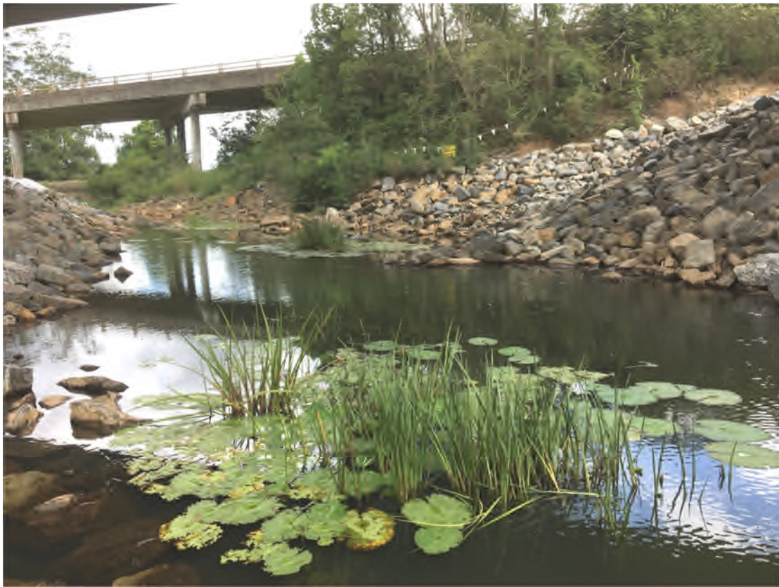
Plate 7: Clumps of Maundia (the sword-leaved aquatic plant) reinstated along Williamson's Creek two years after salvaging Maundia from the creek prior to construction of a new bridge and stabilisation of the creek banks.
