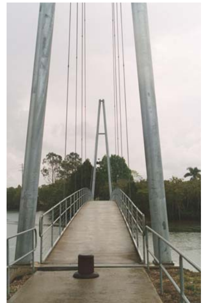
Pedestrian Bridge at Newee Creek
