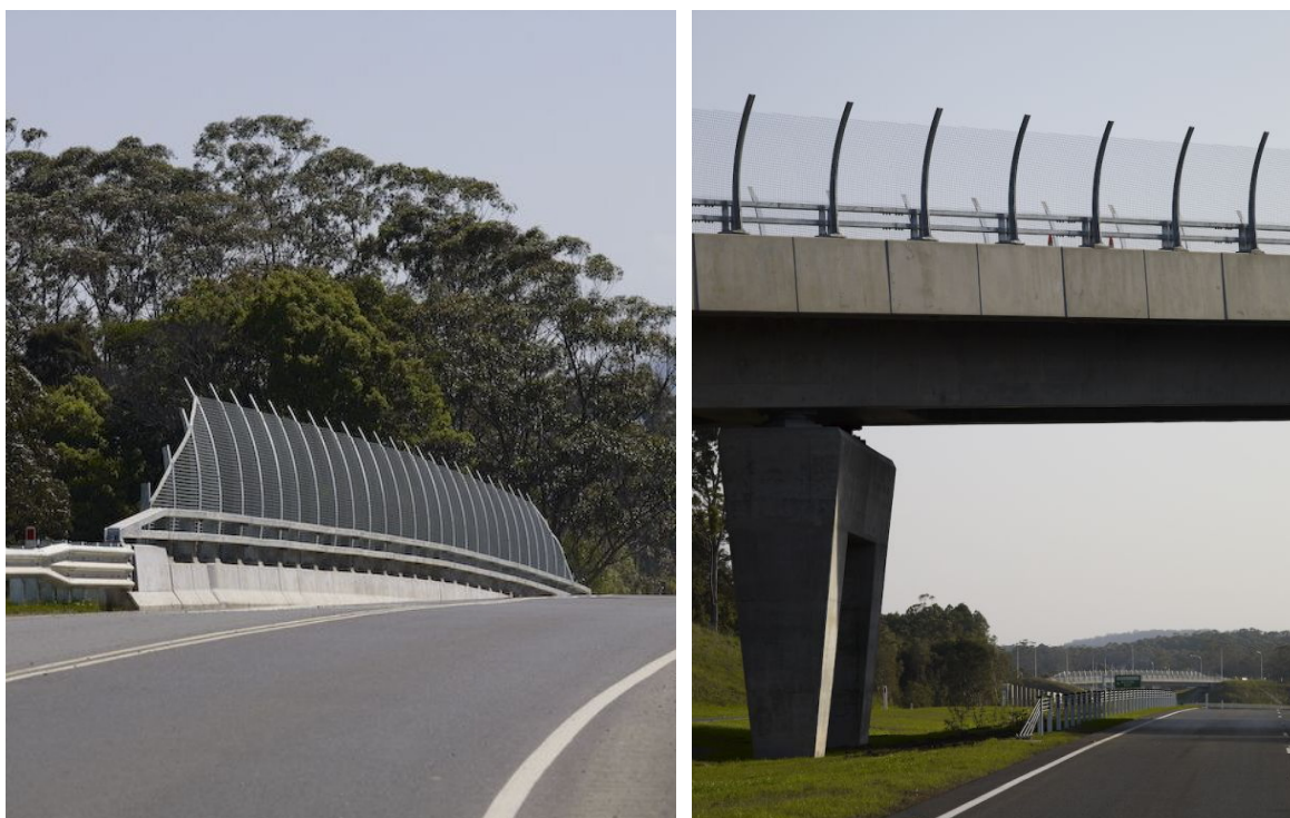
Bridge parts including safety screens and pier junctions in the recently completed Bonville project illustrate well considered junctions and detailing Photos by Brett Boardman
