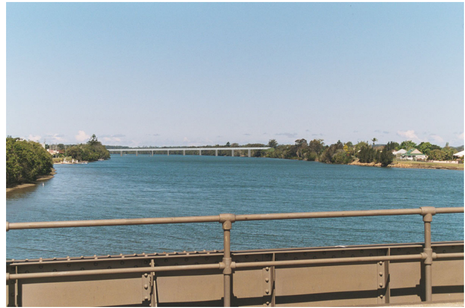
Artist's impression of potential view from Macksville traffic bridge looking east towards proposed bridge over Nambucca River
