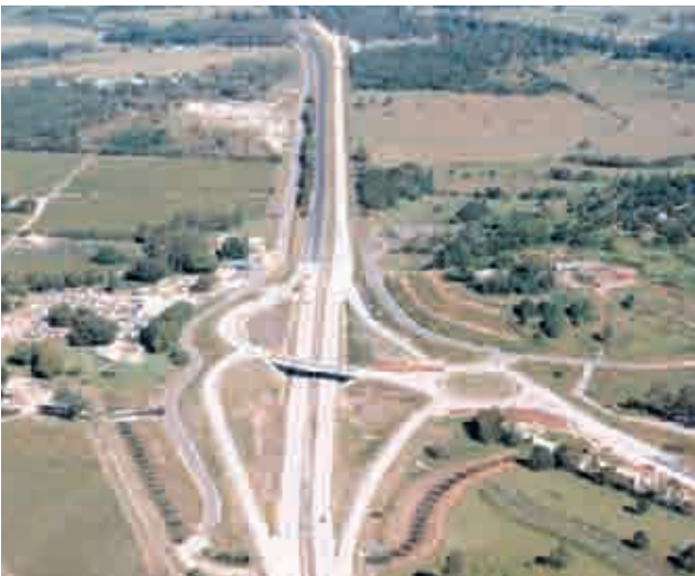
Figure 2: Dual carriageway highway with service road
