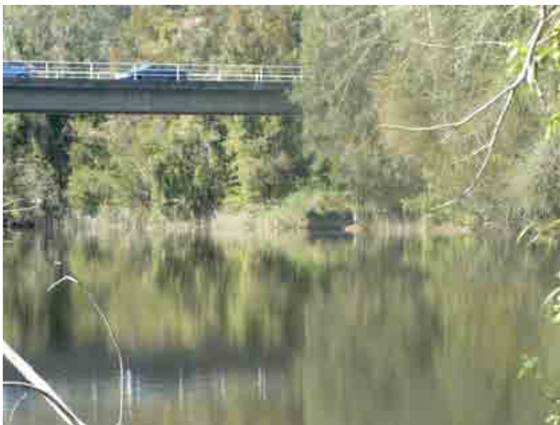
■ Plate 3-13 Warrell Creek downstream
