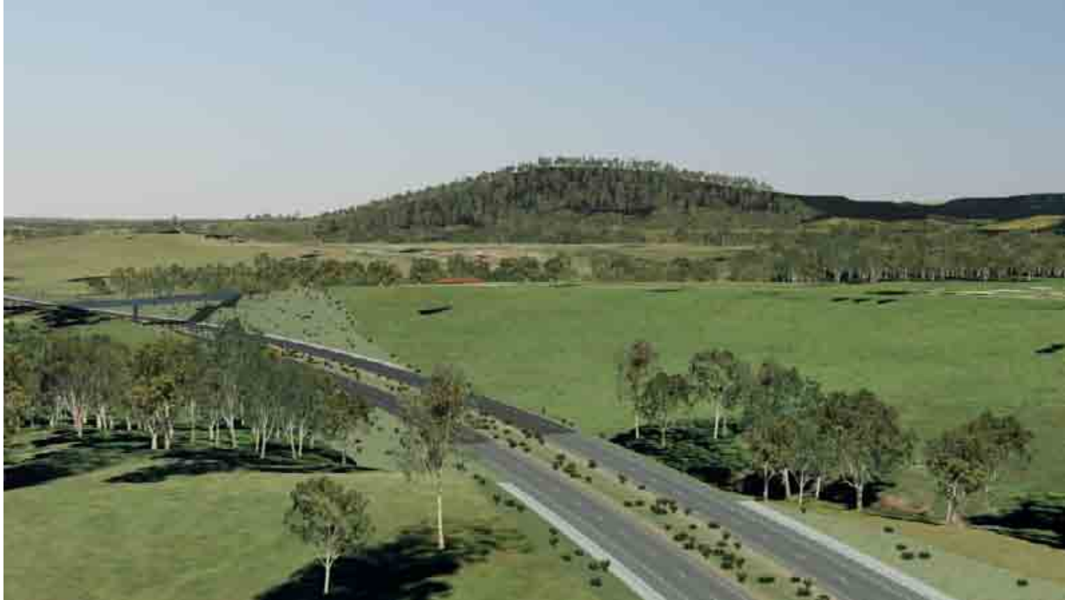
At Rosewood Road the dwellings are situated higher than the road and do not receive the maximum benefit from a noise wall.
