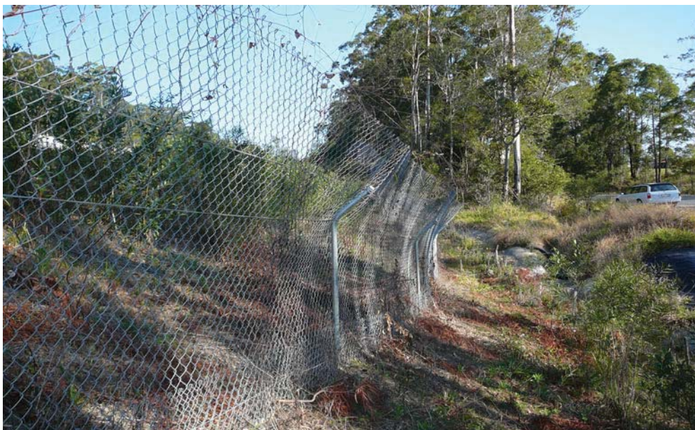
Fig 1. Koala Floppy top fencing installed on the Pacific Highway Bonville Upgrade- shown to be effective at preventing koalas accessing the highway.
