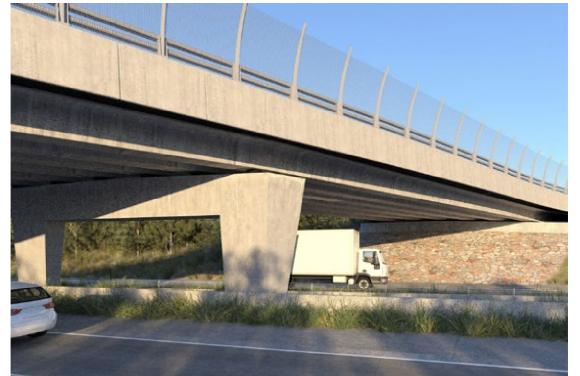
Fig.v Artist impression of tapered median pier at the Broadwater overbridge subject to further design
