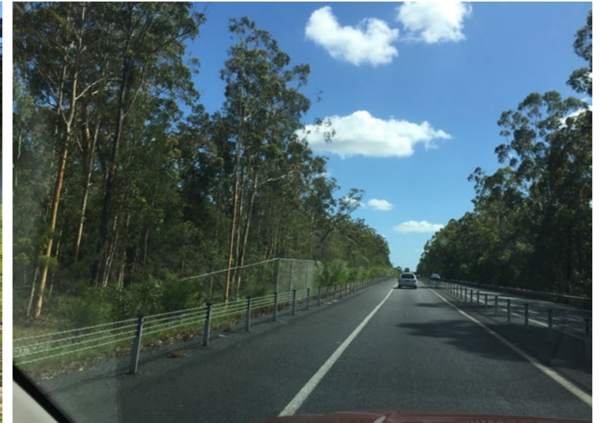
Fig.8.30 Security fencing and wire rope safety barrier
