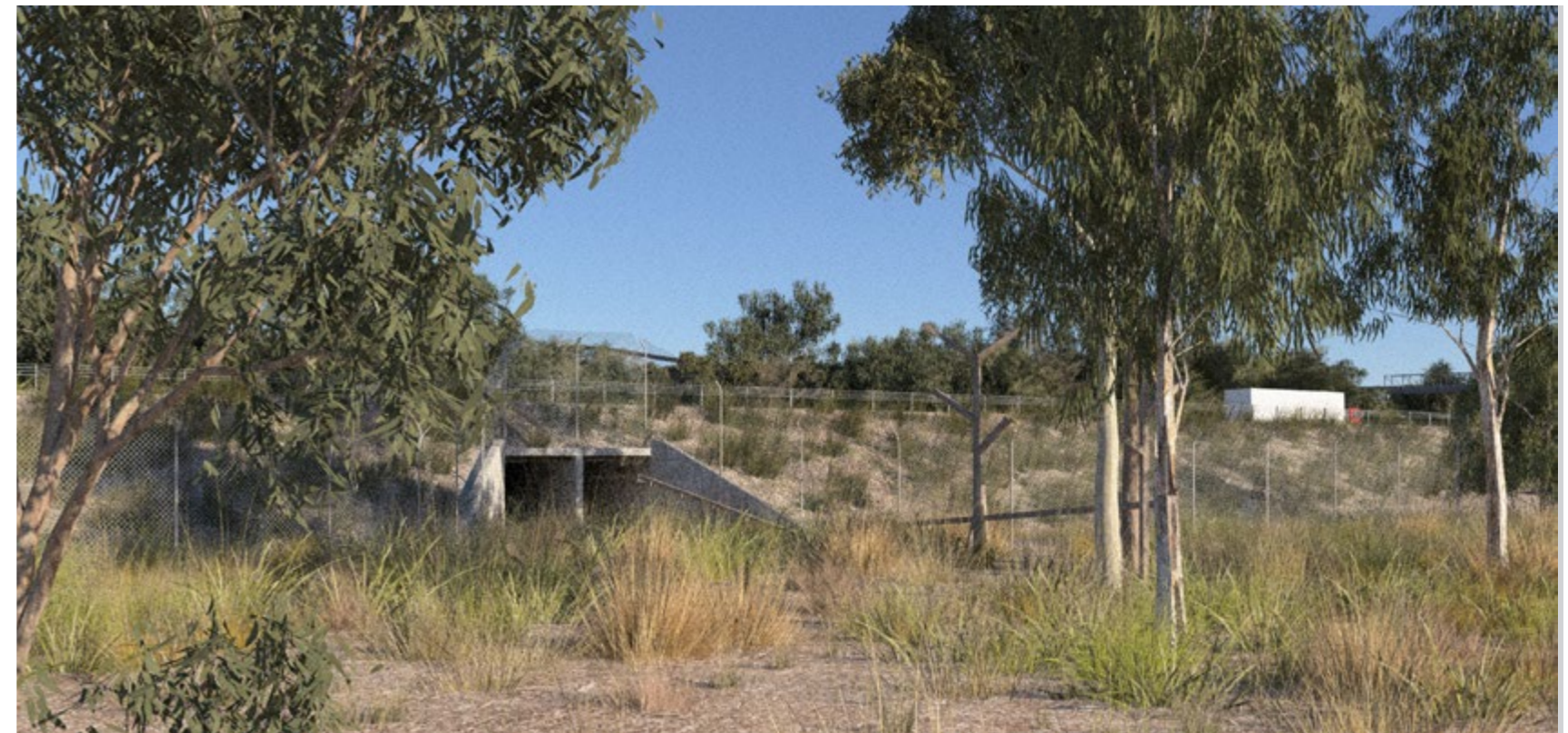
Fig.12.0 Artist impression of fauna culvert with fauna furniture, Landscape shown at full maturity, subject to further design
