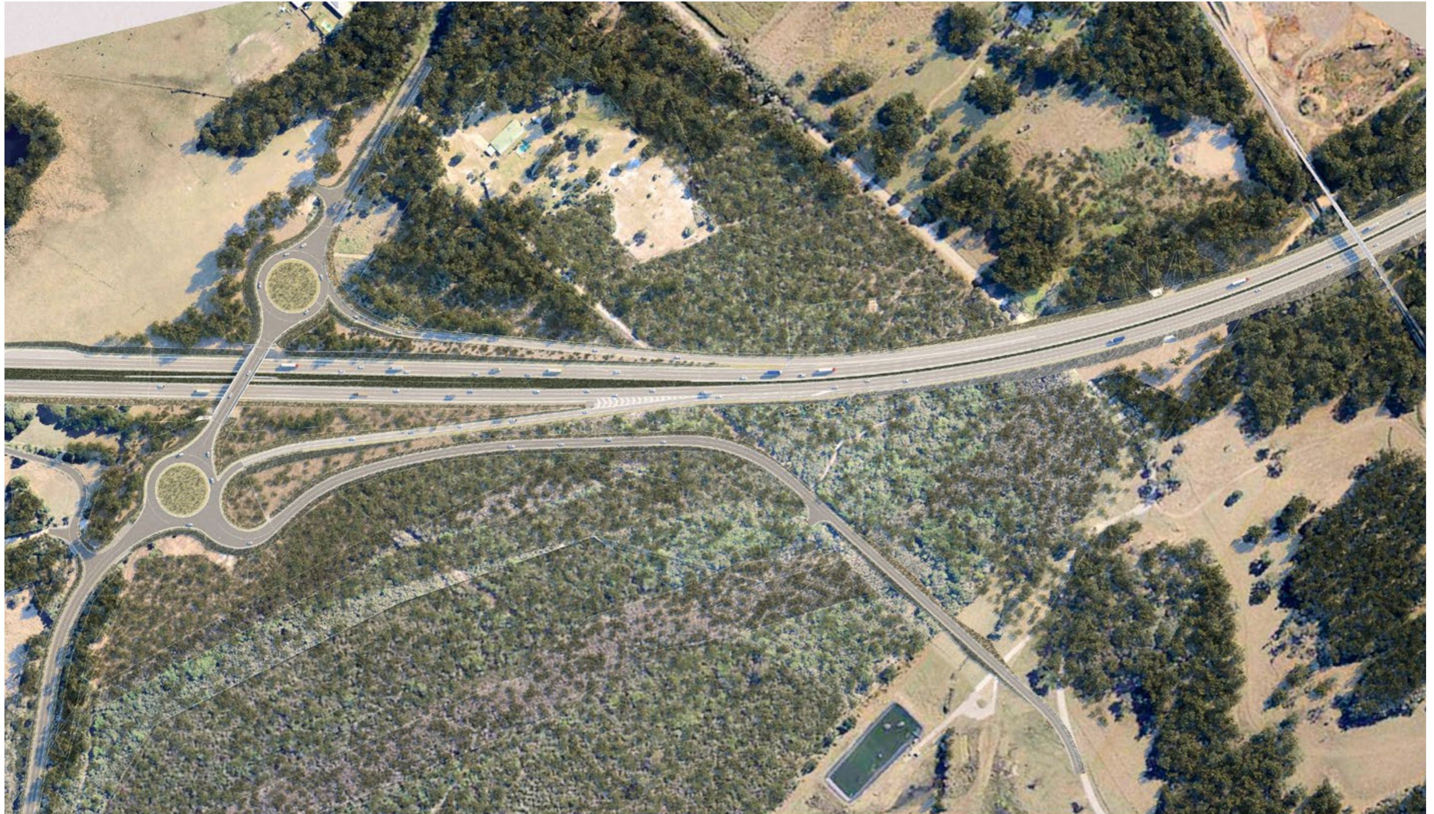
Fig.8.24 Artist impression of aerial view of sugar cane conveyor bridge and its relationship to the Broadwater Interchange. Landscape shown at full maturity. Shared path is subject to further consultation and design development.
