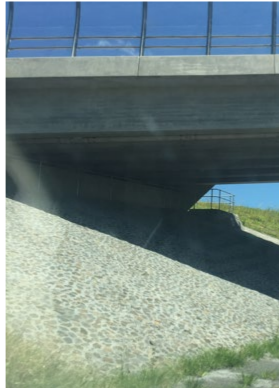
Fig.8.9 Existing abutment
