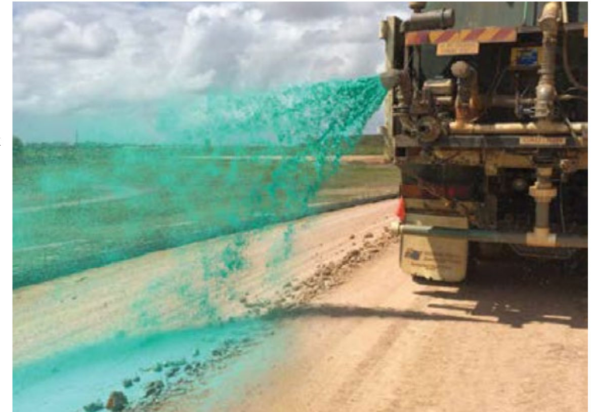
Fig.9.9 Water cart application of a tackifier.(Photo: Vital Chemical Pty Ltd)
