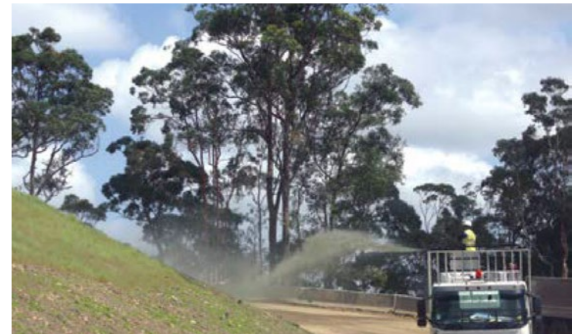
Fig.9.10 Standard Hydromulch being applied to a batter on the Hunter Expressway.
