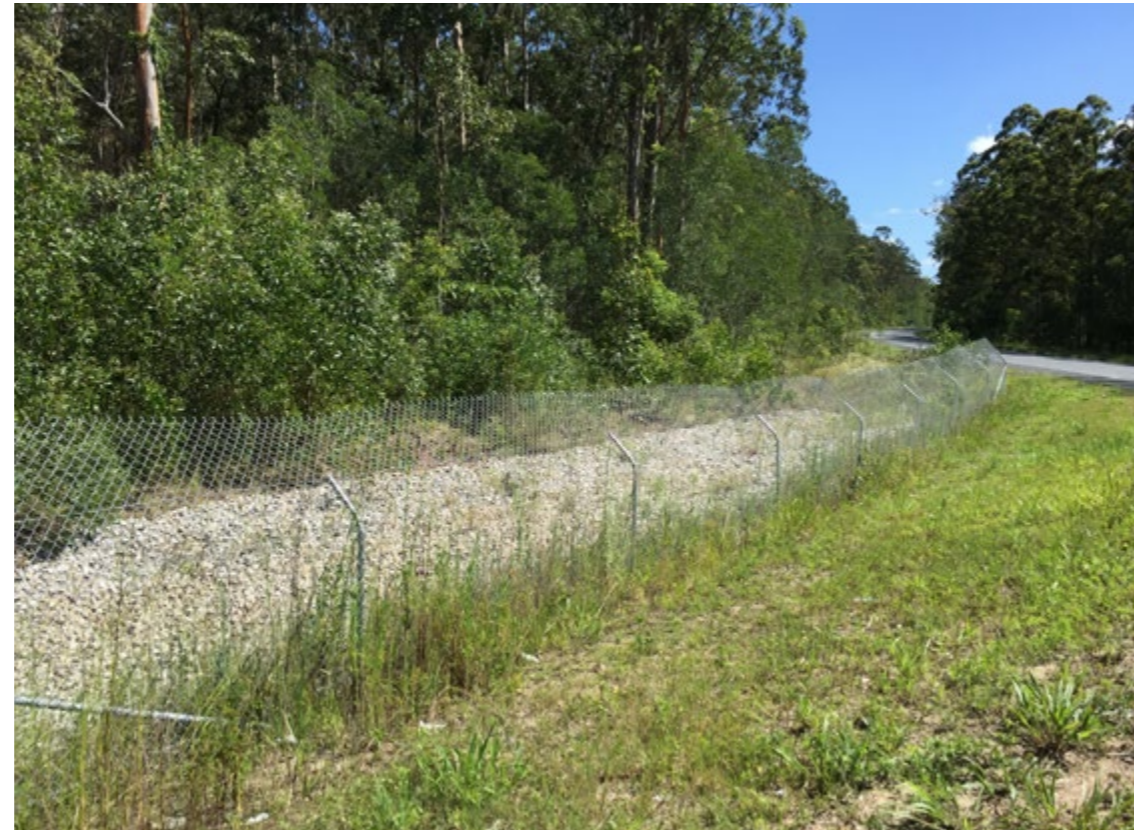
Fig.8.29 Typical fauna fence, fauna fence style under review
