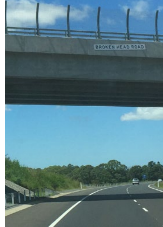
Fig.8.10 Existing bridge parapet and girder
