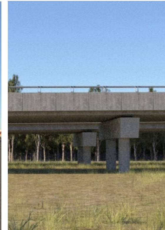
Fig. 8.23 Piers and headstock
