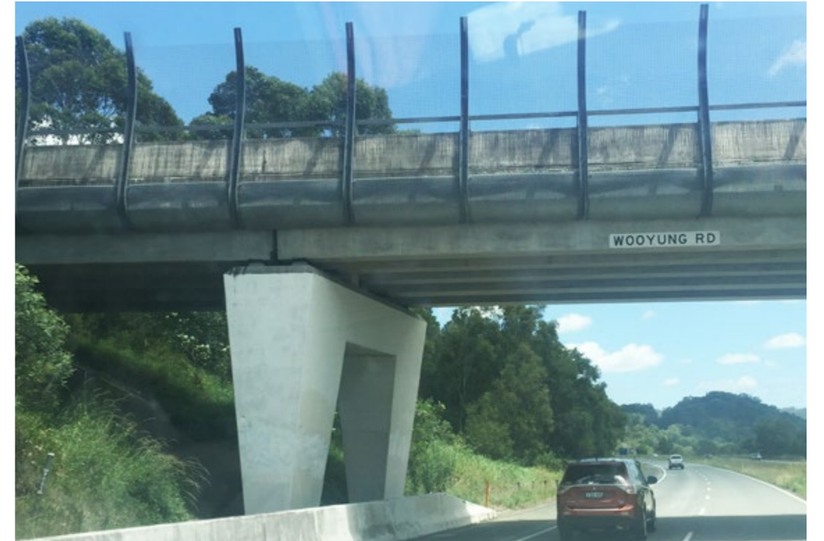
Fig.iv Existing Wooyung Road overbridge with tapered median pier
