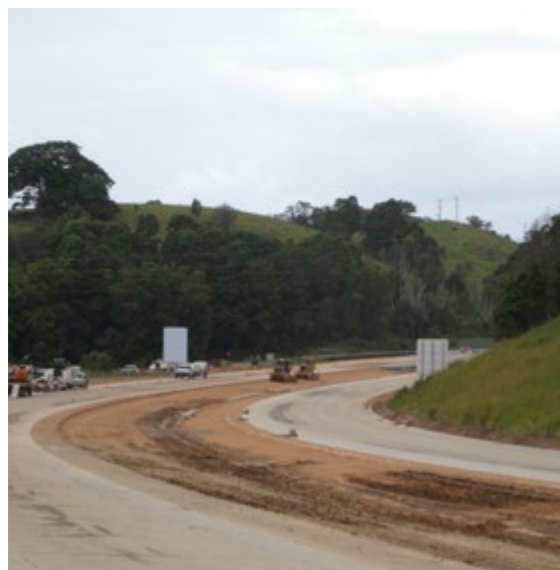
Fig.10.1 Cleared median awaiting seeding
