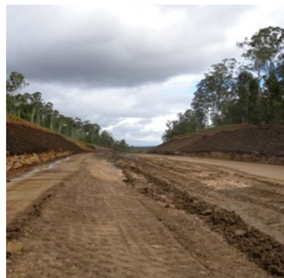
Fig.10.2 Cut batter before roadwork and planting
