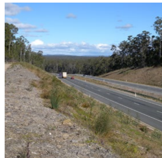
Fig.10.4 Cut batter with new planting growth 15 months after seeding
