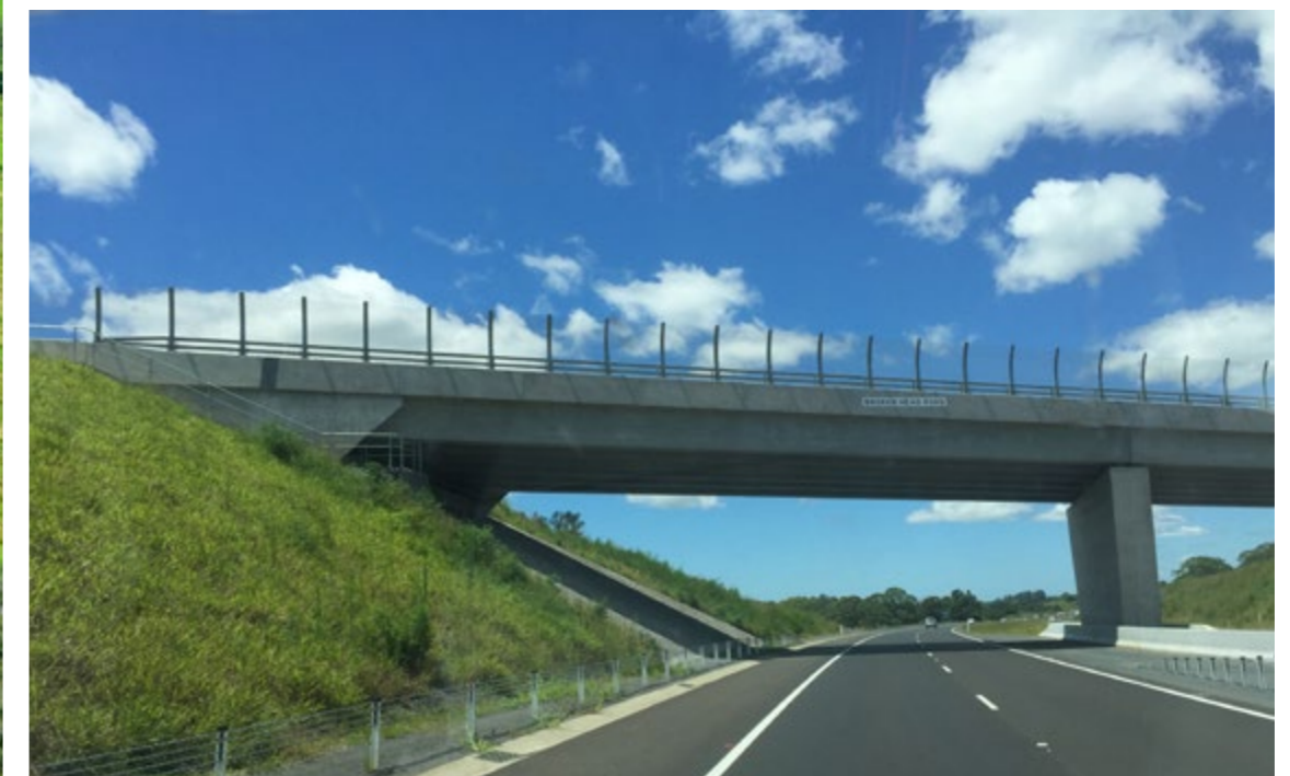
Fig 6.3 Existing bridge, (Image source: ACJV)
