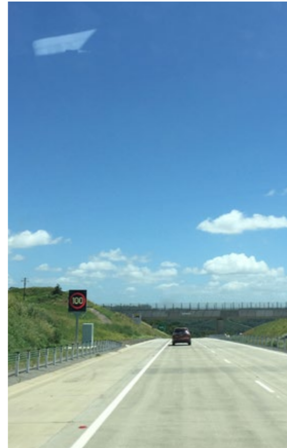
Fig.5.2 Existing Pacific Highway road edge. (Image source: ACJV)
