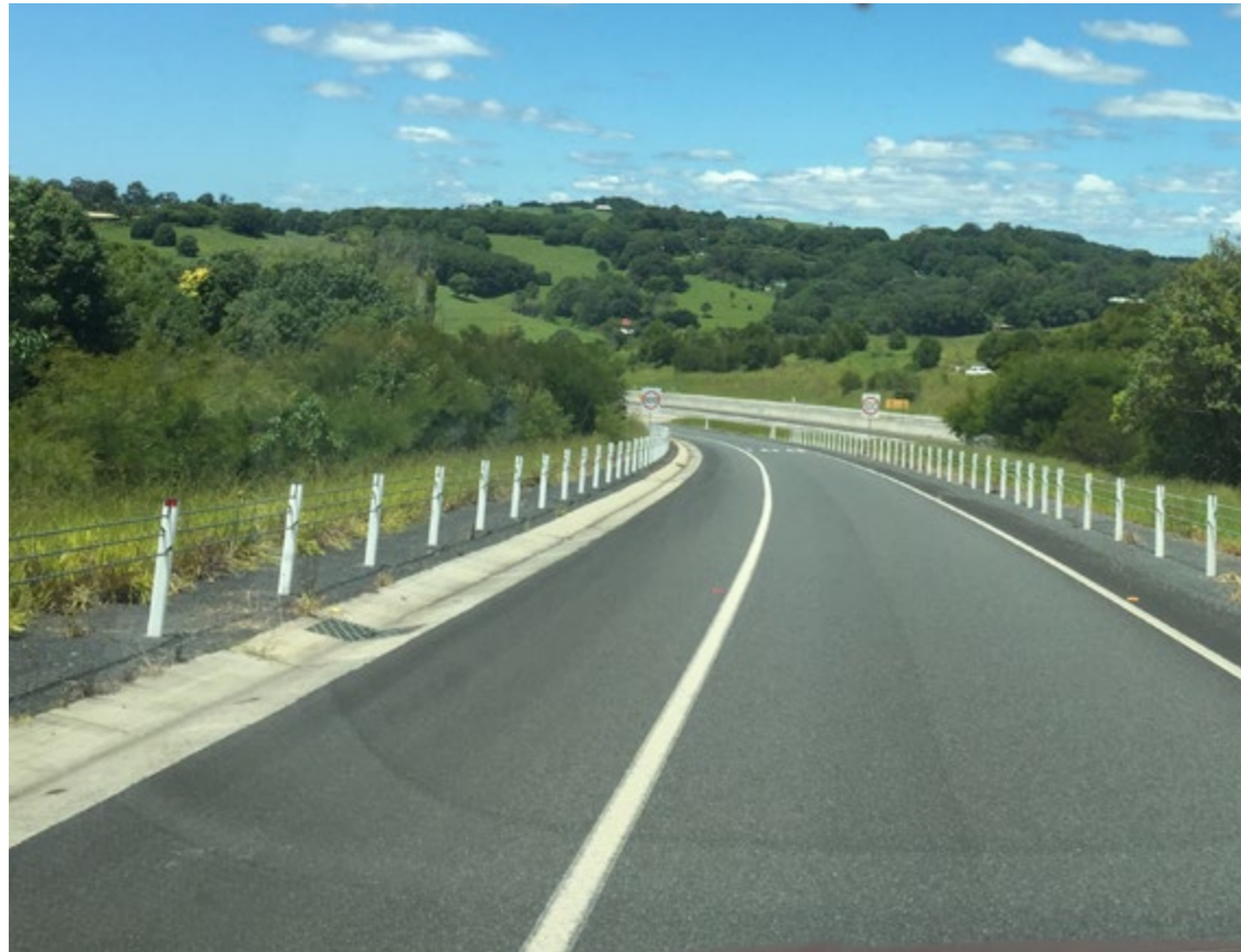
Fig.5.1 Existing Pacific Highway road alignment and character. (Image source:ACJV)
