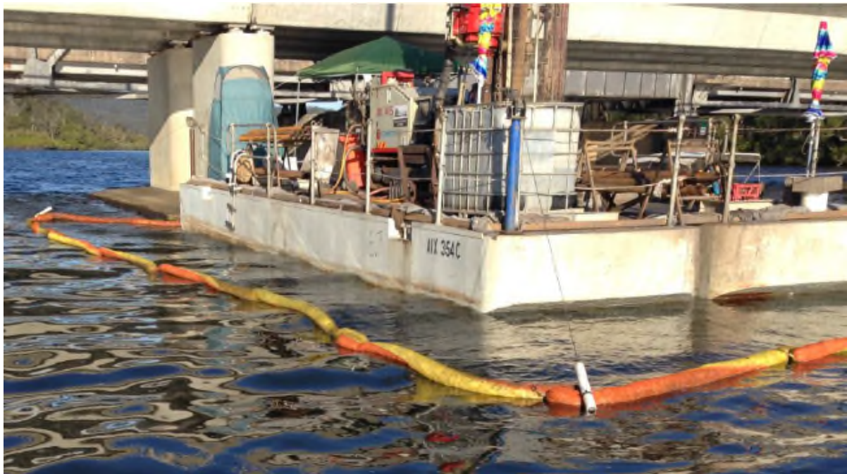
Figure 3.2 Boom placement following implementation of PVC sliders
