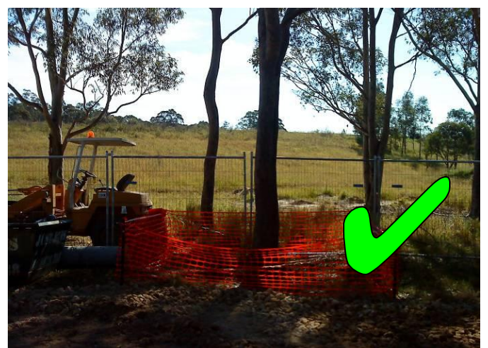
Figure 5: Tree protected via fencing with no materials stored within the drip line.
