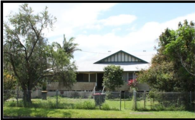
Convent within Harwood village. Section 5 (Portion B)
