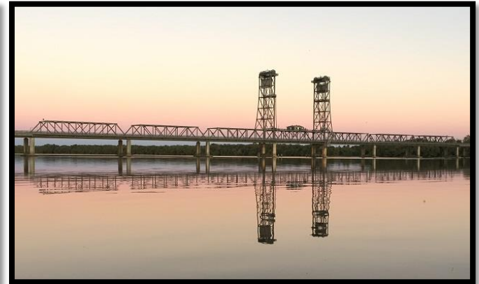
Harwood Bridge, Harwood. Section 5 (Portion B)
