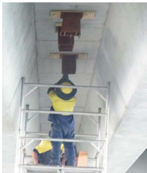
Plate 3.8 Installation of bat boxes beneath Mororo Bridge (Source: D Andrighetto)
