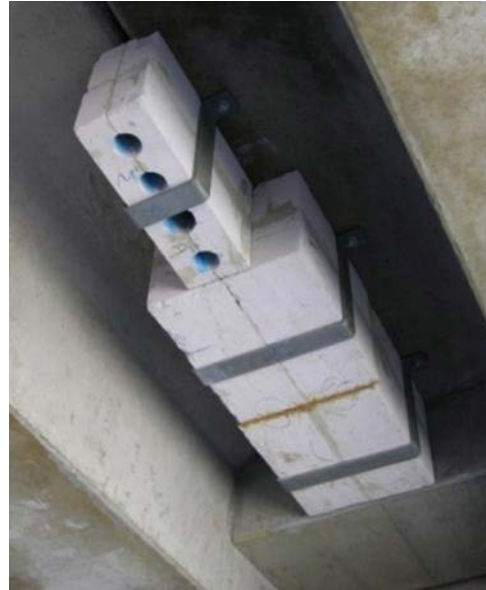
Plate 3.10 Lightweight concrete beneath bridge (Source: N Williams)
