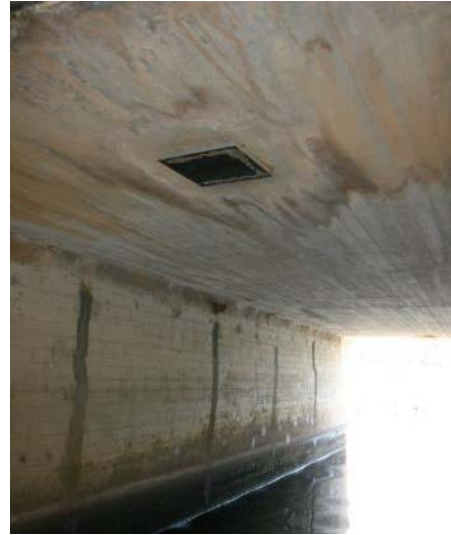
Plate 3.2 Plywood blocking a lift hole at Halfway Creek culvert (Source: V Silver)
