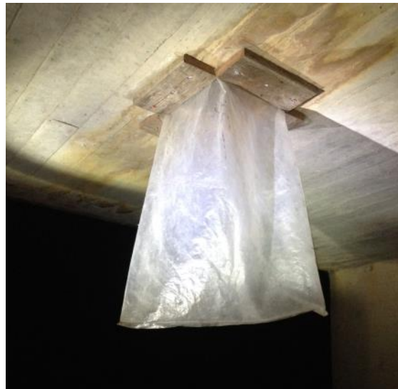
Plate 3.2 Plywood blocking a lift hole at Halfway Creek culvert (Source: V Silver)
