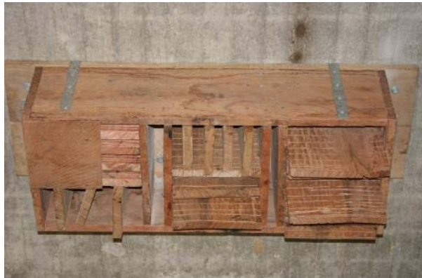
Plate 3.12 Lattice style bat box under Halfway Creek Bridge (Source: V Silver)
