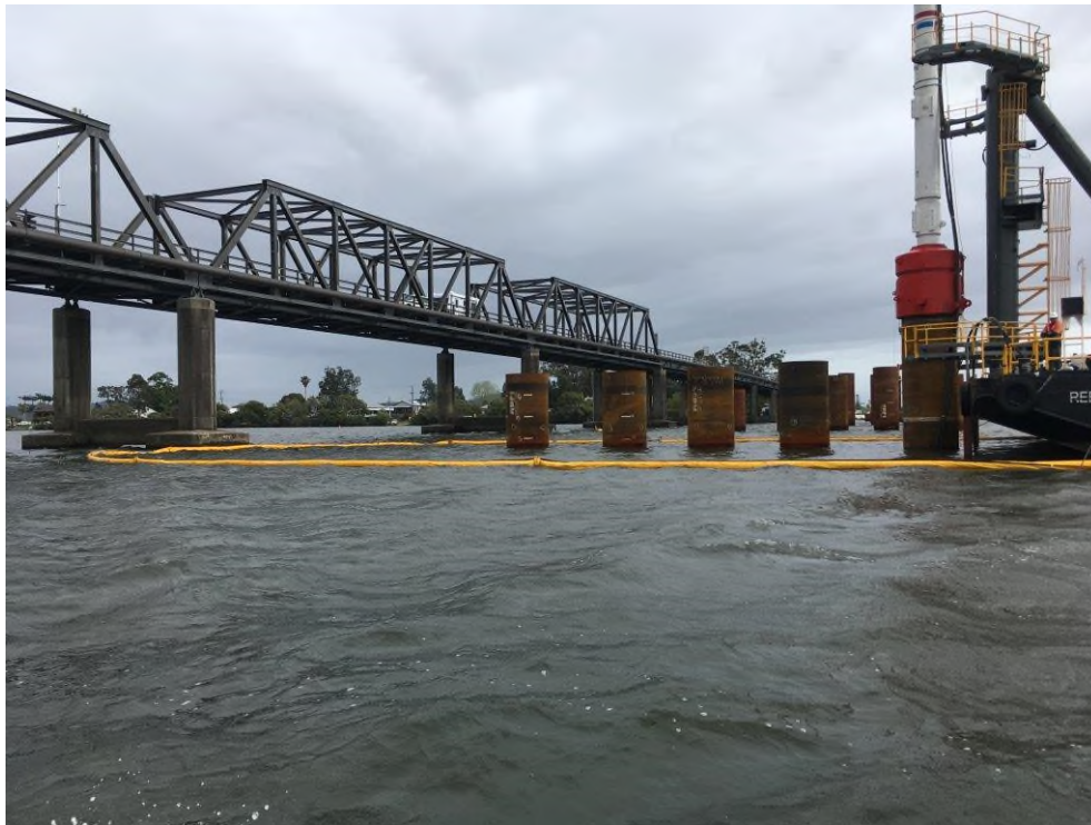
Figure 3 – spill containment boom deployed to manage works in river
