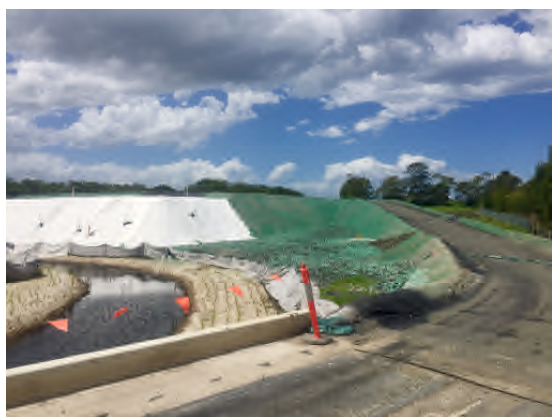
Figures 2 Erosion and sediment controls implemented prior to shutdown for OPP Spawning Season (October to April)
