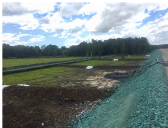
Figures 2 Erosion and sediment controls implemented prior to shutdown for OPP Spawning Season (October to April)
