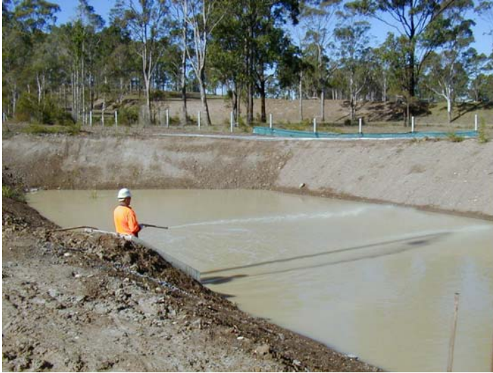
Figure 1. Application to a sediment basin allows faster settling of sediments and improvements to water quality prior to discharge.
