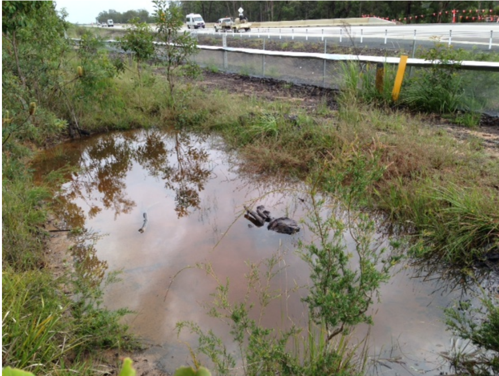
Photos: frog habitat ponds installed near CH19100 full following extended heavy rainfall (20 March 2017)
