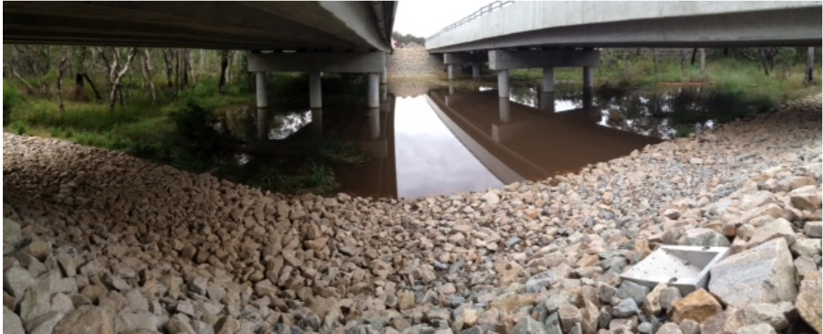
Photo: Wells Crossing June 2017 following removal of temporary access platform between the two bridges in May 2017. Note retention of riparian vegetation and trees immediately adjacent to both the northbound and southbound bridges
