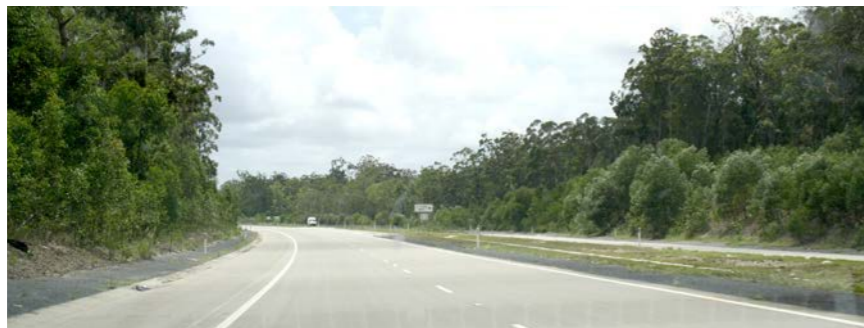
Plate 5-18: View north travelling on the Pacific Highway through landscape character precinct 34 at the Devils Pulpit upgrade
