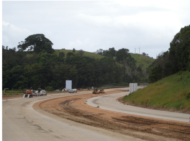
Plate 8-2: Ballina Bypass, February 2011
