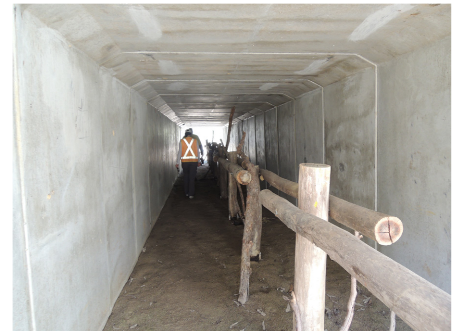
Figure 8-6: Example of fauna furniture inside culvert
