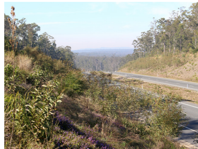
Plate 8-8: Glenugie Upgrade, August 2013
