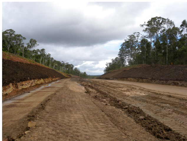
Plate 8-6: Glenugie Upgrade, April 2011
