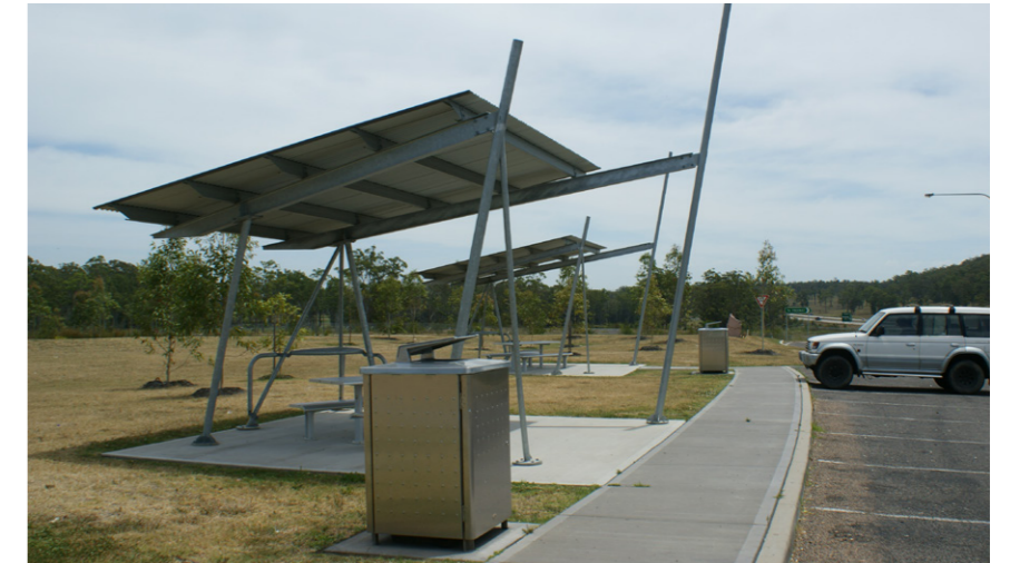
Plate 8-1: Picnic shelters at the Hunter Expressway westbound rest area
