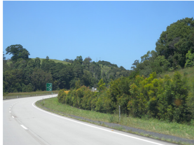
Plate 8-3: Ballina Bypass, January 2015
