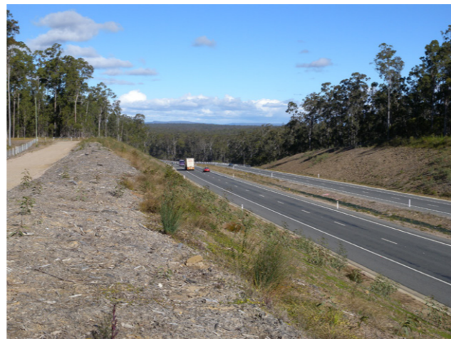
Plate 8-7: Glenugie Upgrade, July 2012
