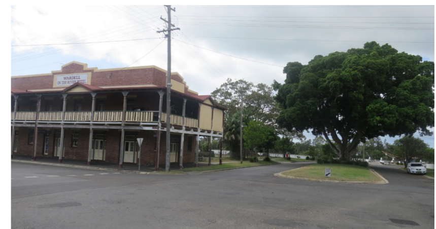
Figure 15: Main street of Wardell with hotel and feature Fig trees in the foreground and Richmond River beyond, Character Precinct 51
