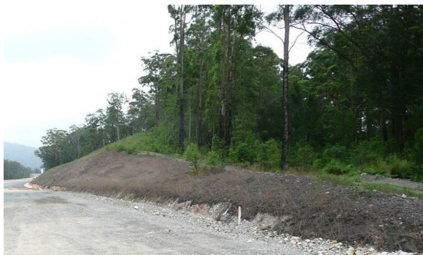
Figure 65: Batter stabilisation
