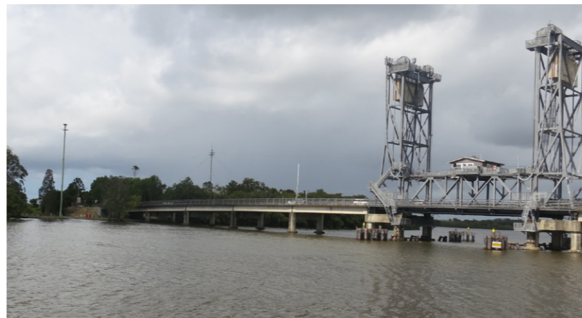
Figure 22: View of Richmond River and existing bridge at Wardell
