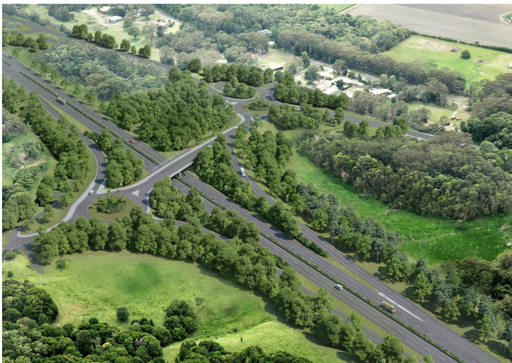
Figure 1: The design on the approach to Coolgardie Interchange signals the entry in to Wardell township (Artists impression subject to further design development. Landscape shown at maturity. Inclusion of shared path subject to further consultation)
