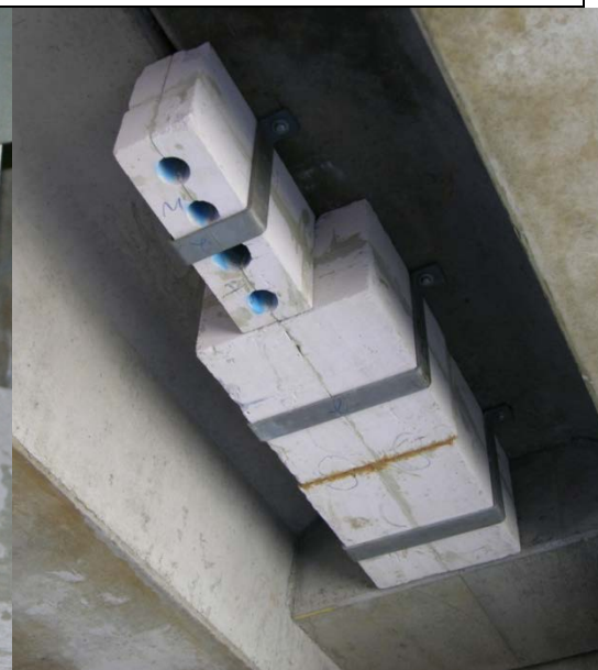
Plate 3.10 Light weight concrete blocks with drill holes secured beneath bridge (Source: N. Williams)
