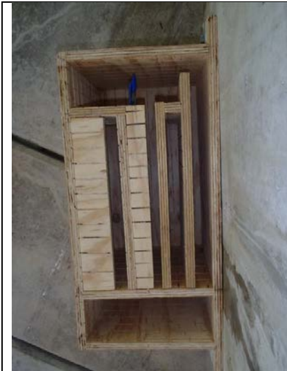
Plate 3.11 Lattice style bat box beneath Myott Bridge (Source: A. Lloyd)
