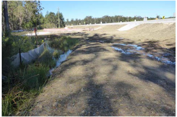
Mt-2.1 Looking SW at damming effect of highway, bank and sediment fence June 2016
