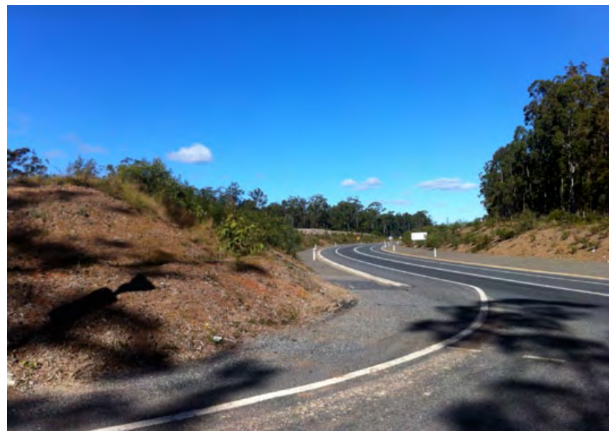
Plate 4.2: Recently completed Glenugie upgrade, typical of Section 2. Landscape character precinct 8 (refer Figure 4.1).
