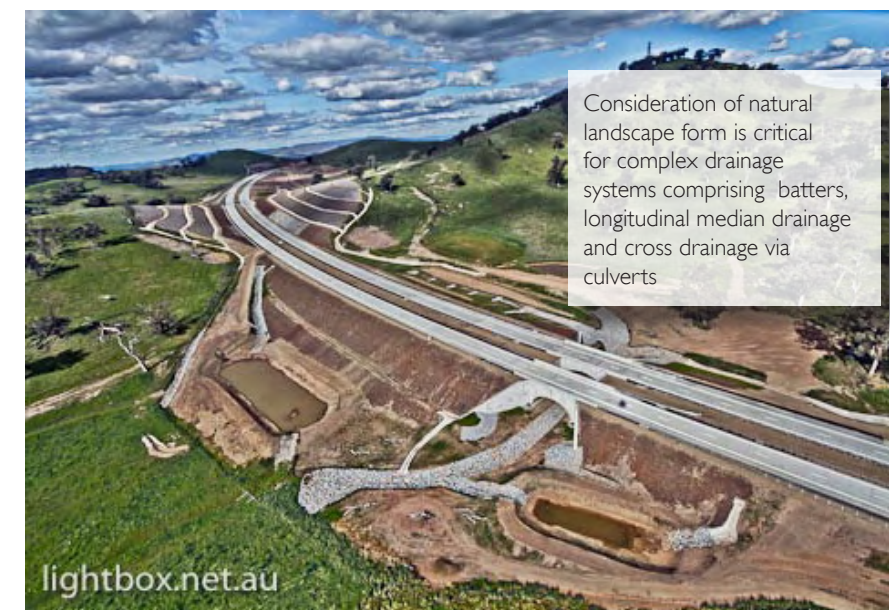
Plate 3.2: Complex drainage system at Hume Highway Woomargama Bypass (Source: Lightbox/ HHWA)
