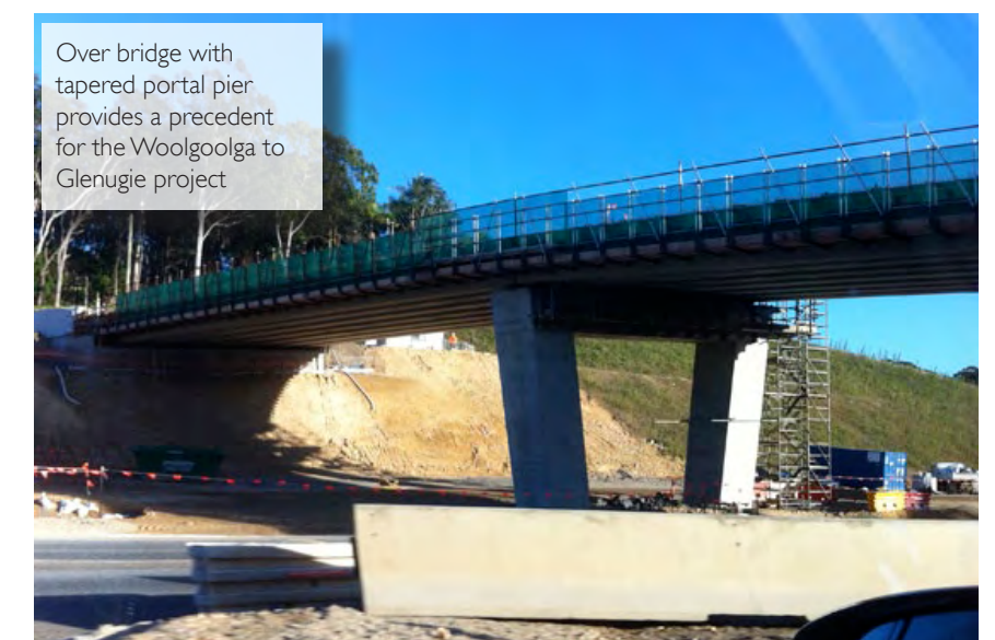
Plate 3.1: Similar overbridge under construction on the Sapphire to Woolgoolga project
