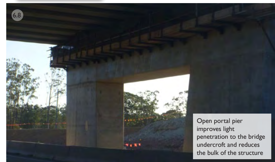
Plate 6.6: Twin Bridges on Hume Highway Woomargama Bypass at Mountain Creek
