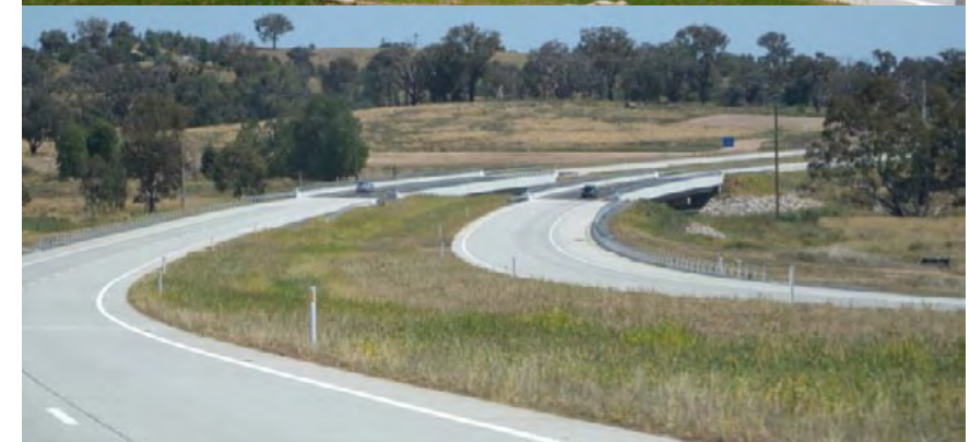
Plate 6.18: Hydroseeding of median invert and direct drill seeding of median batters on the Hume Highway Woomargama Bypass at time of installation and after 2 seasons (bottom) (Source: Roads and Maritime and SMM)
