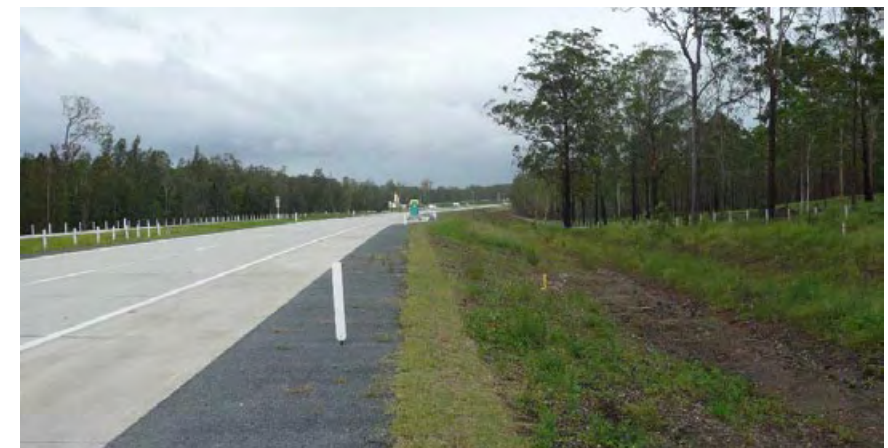
Plate 6.19: Turf strip installed along verge edges at Pacific Highway Kempsey Bypass (Source: Roads and Maritime)
