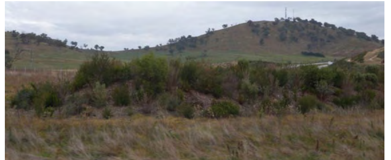
Plate 6.10: Headlight glare screening mound on Hume Highway Woomargama Bypass
