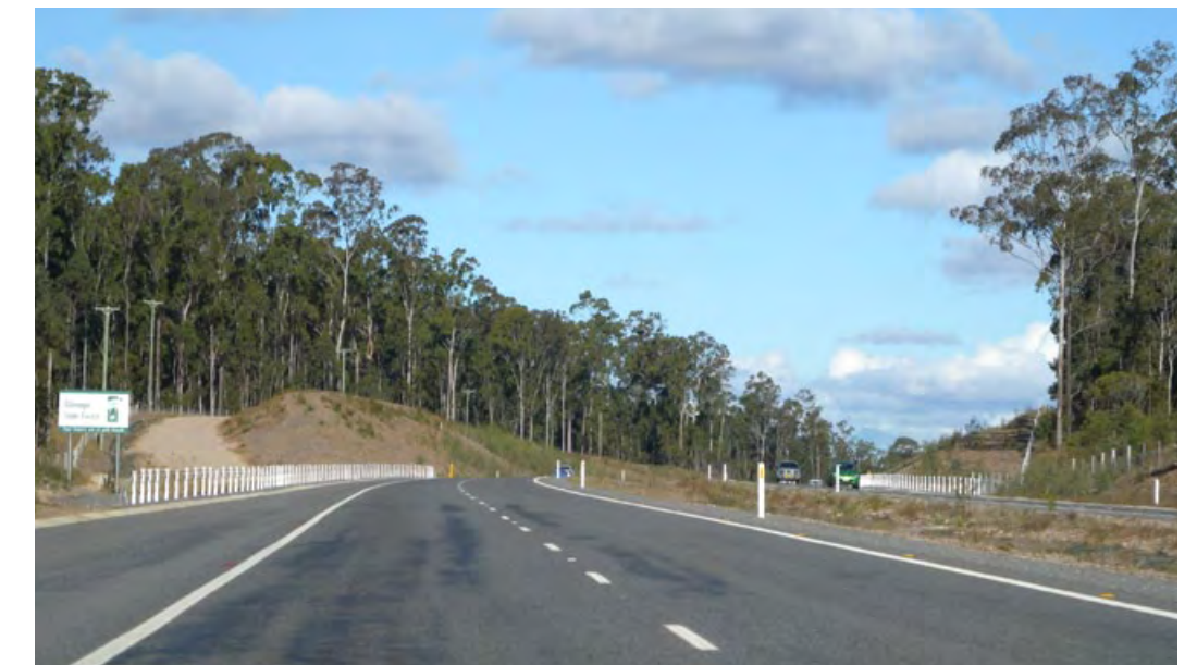
Plate 2.6: Pacific Highway, Glenugie upgrade
