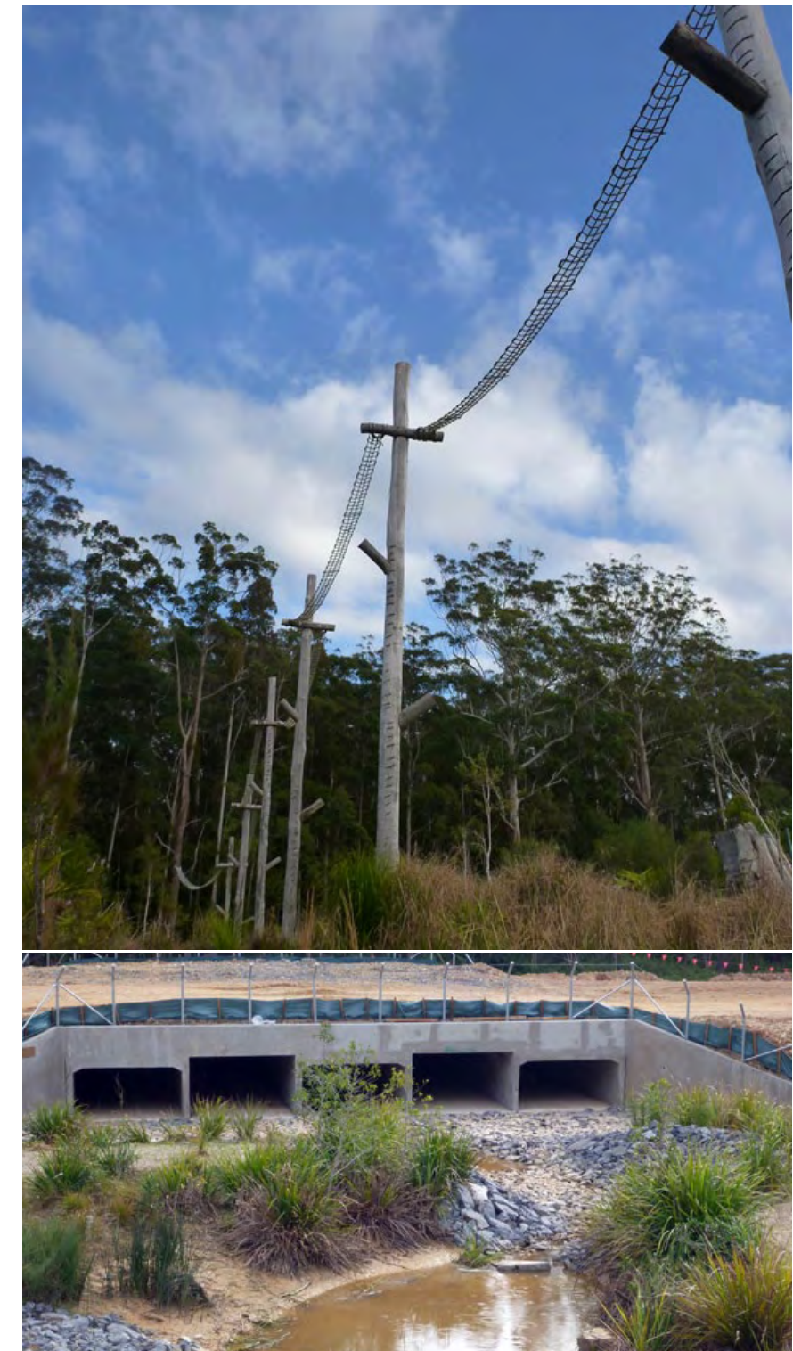
Plate 6.13: Fauna culvert crossing and mini wetland habitat provision on the Pacific Highway upgrade, Sapphire to Woolgoolga (Image source SMM)
