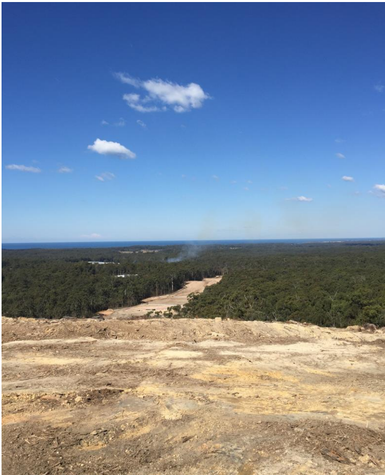
Looking south at earthworks near Hawthorn Close at Corindi Beach (August 2015)
