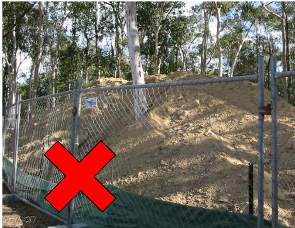
Figure 4: Spoil stored within the drip line of trees.
