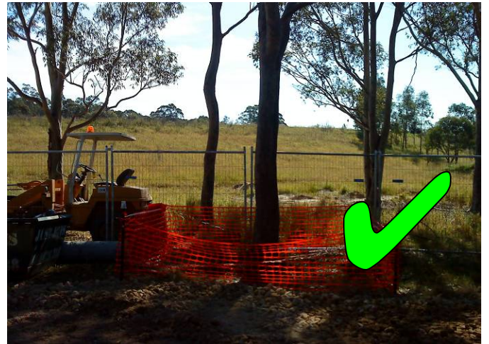
Figure 5: Tree protected via fencing with no materials stored within the drip line.
