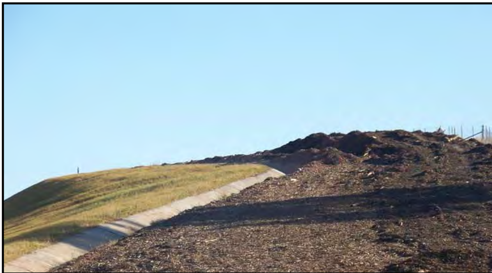
Plate 7: Mulch being placed as batter erosion control. Mulch should not be applied in layers more than 100 mm thick for surface stabilisation.
