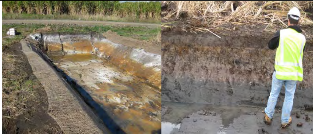
Photo 1 – Temporary treatment area
