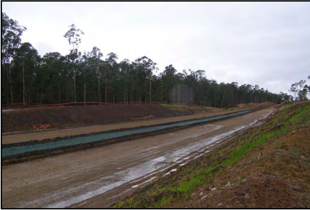
Plate 8: Site showing recent application of a mulch/topsoil mix on batters (40% mulch to 60% topsoil). Mulch mixes are used to provide temporary stabilisation to prevent the loss of topsoil from batters in heavy rainfall events. Mulch use is also shown as a mounded sedimentation control to prevent sediment entering the median drain.
