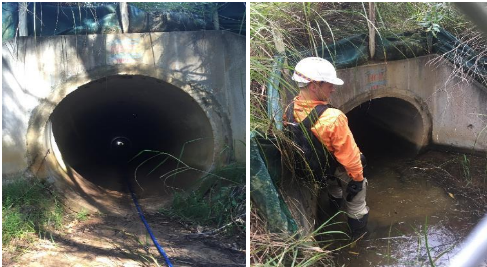
Plate 4: Non-excluded RC pipe #67 featured two eastern horseshoe bats at the summer inspection (L). Approximately 50-300mm of water flowed through the pipe during winter (R).
