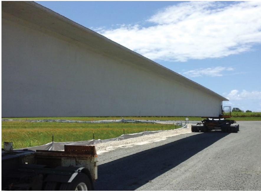
One of 234 girders being delivered to site
