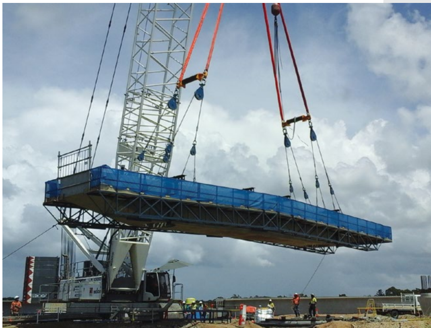
The first of 35 headstocks was installed in February
