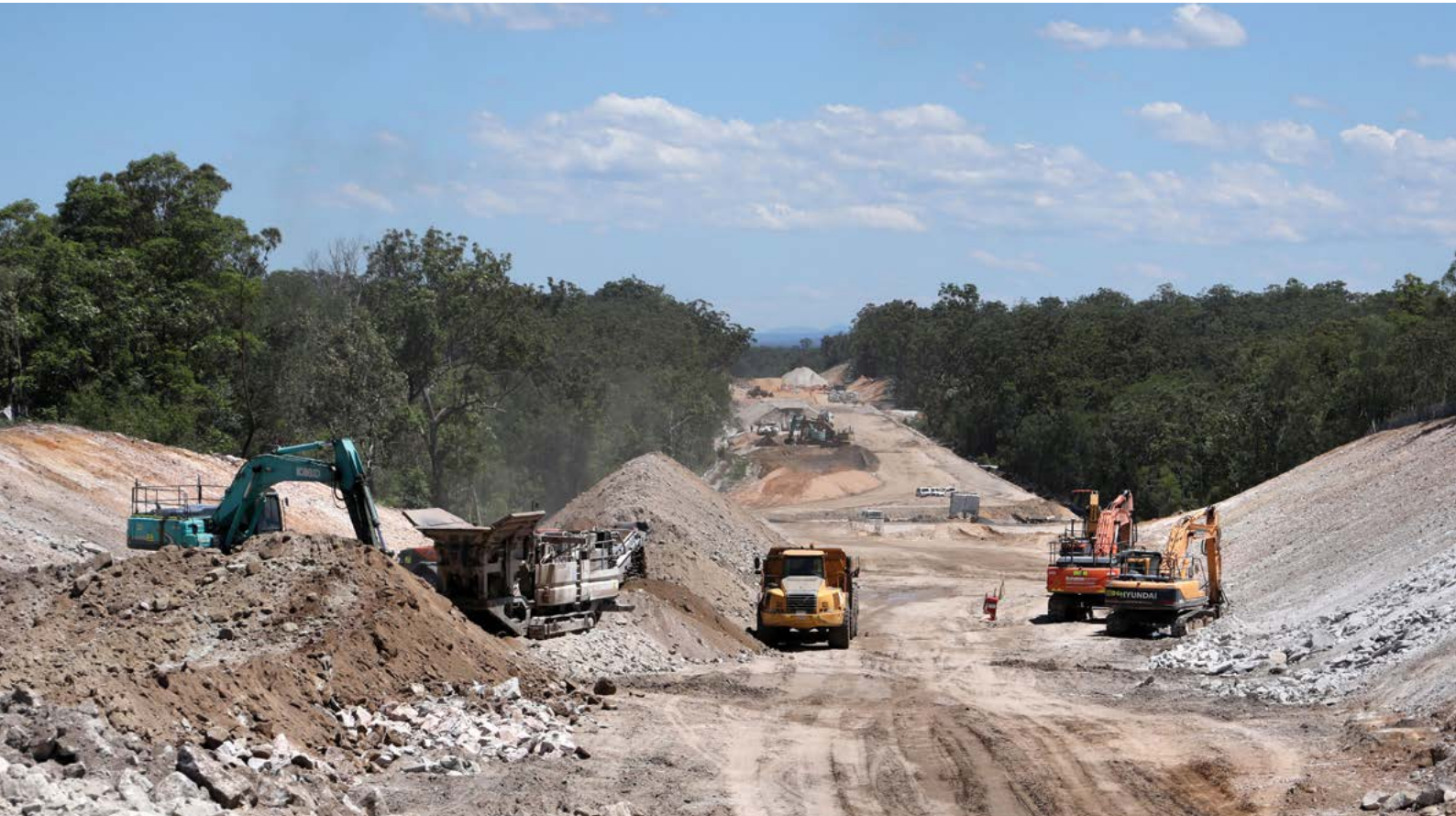
Earthwork between Glenugie and Maclean
