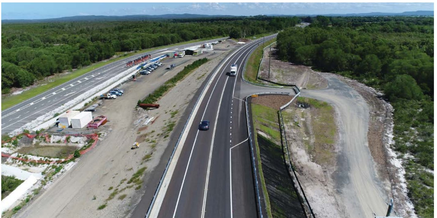
New service road at Broadwater
