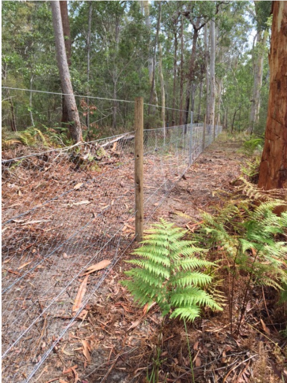
Plate 2. Example of emu exclusion fenced trialled during pre-construction
