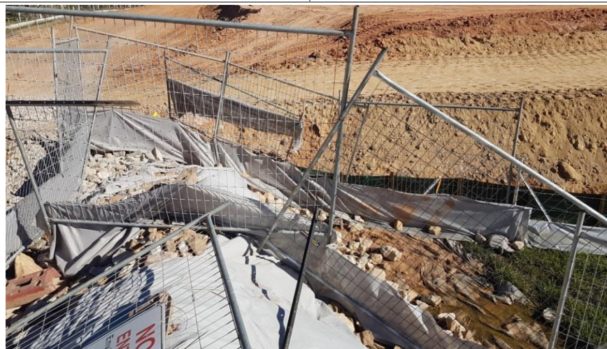
Plate 22 Western batter of haul road.
