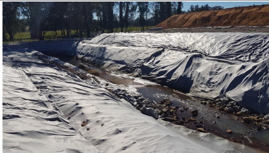
Plate 8 Western end of creek viewed from southern edge.
