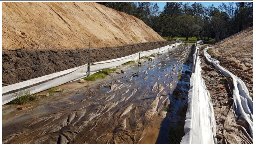
Plate 14 Central section of run viewed from northern edge (looking west).
