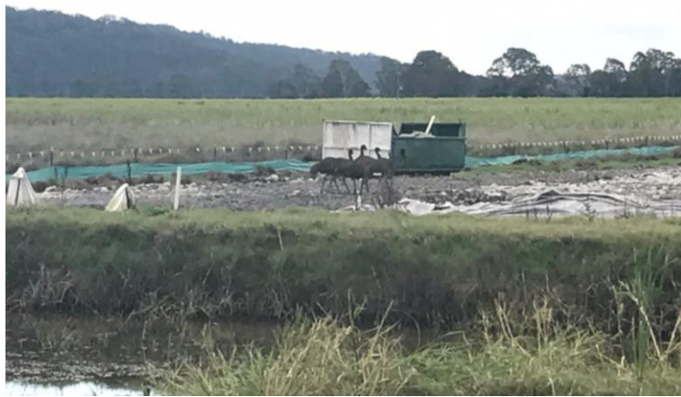
Plate 1: Emus recorded on Shark Creek Bridge piling pad, 3 July 2017. Source: Brenden Bale, Pacific Complete.
