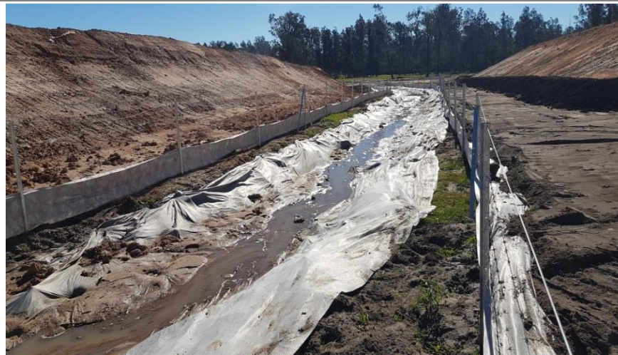
Plate 11 Middle of run viewed from northern edge (looking west).
