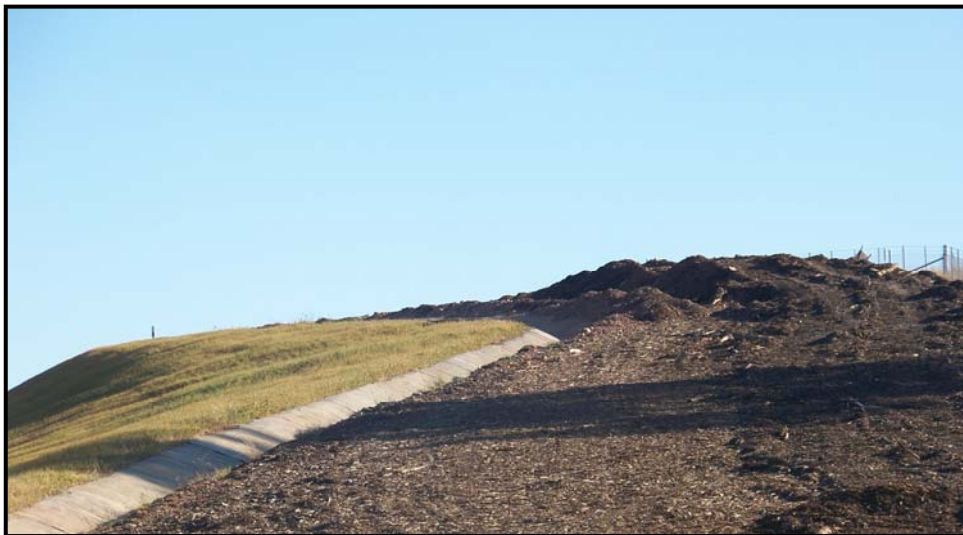
Plate 7: Mulch being placed as batter erosion control. Mulch should not be applied in layers more than 100 mm thick for surface stabilisation.
