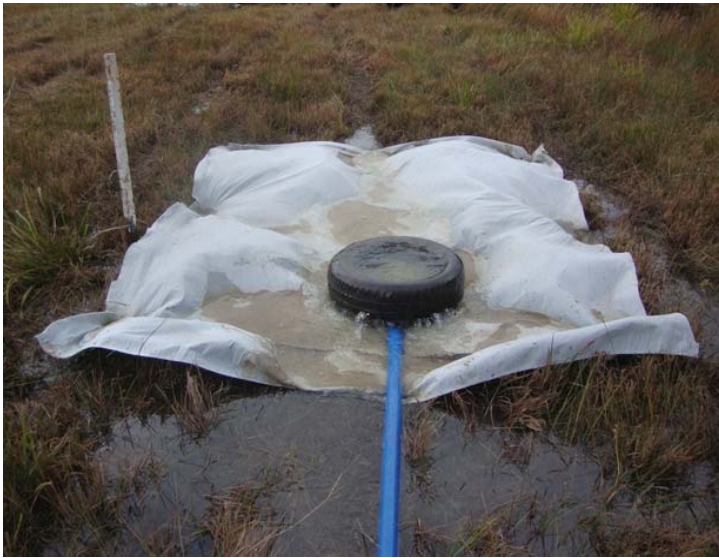
Figure 3. Informal use of bunding and geotextile was assessed as a suitable outlet treatment for scour protection in this example. The use of a tyre provided both energy dissipation for the discharge flow and anchorage for the discharge pipe.
