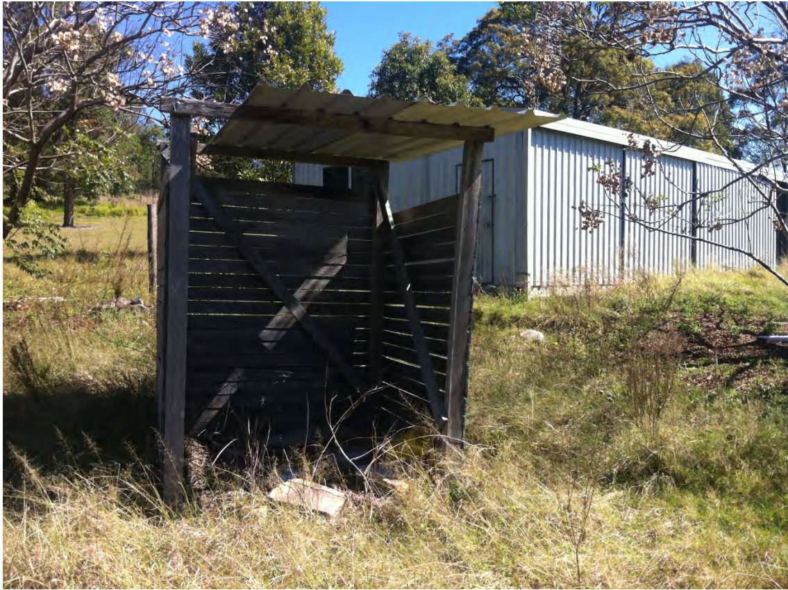
Plate 13 – Small timber structure located to north-east of shed
