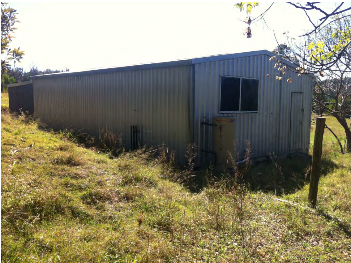
Plate 12 – Southern and eastern sides of shed
