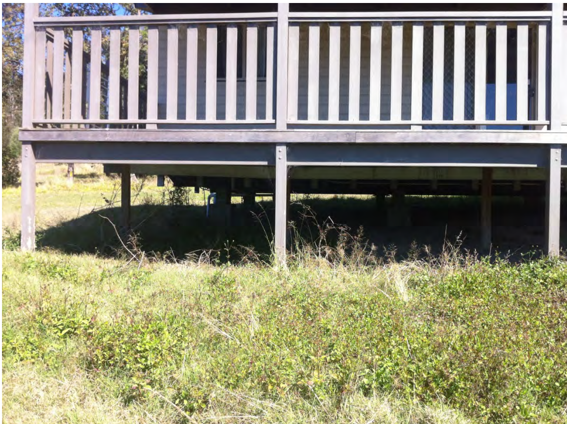
Plate 2 – View of underneath of house
