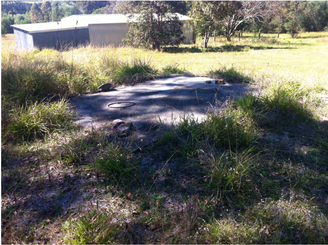
Plate 21 – Concrete slabs to south-west of shed
