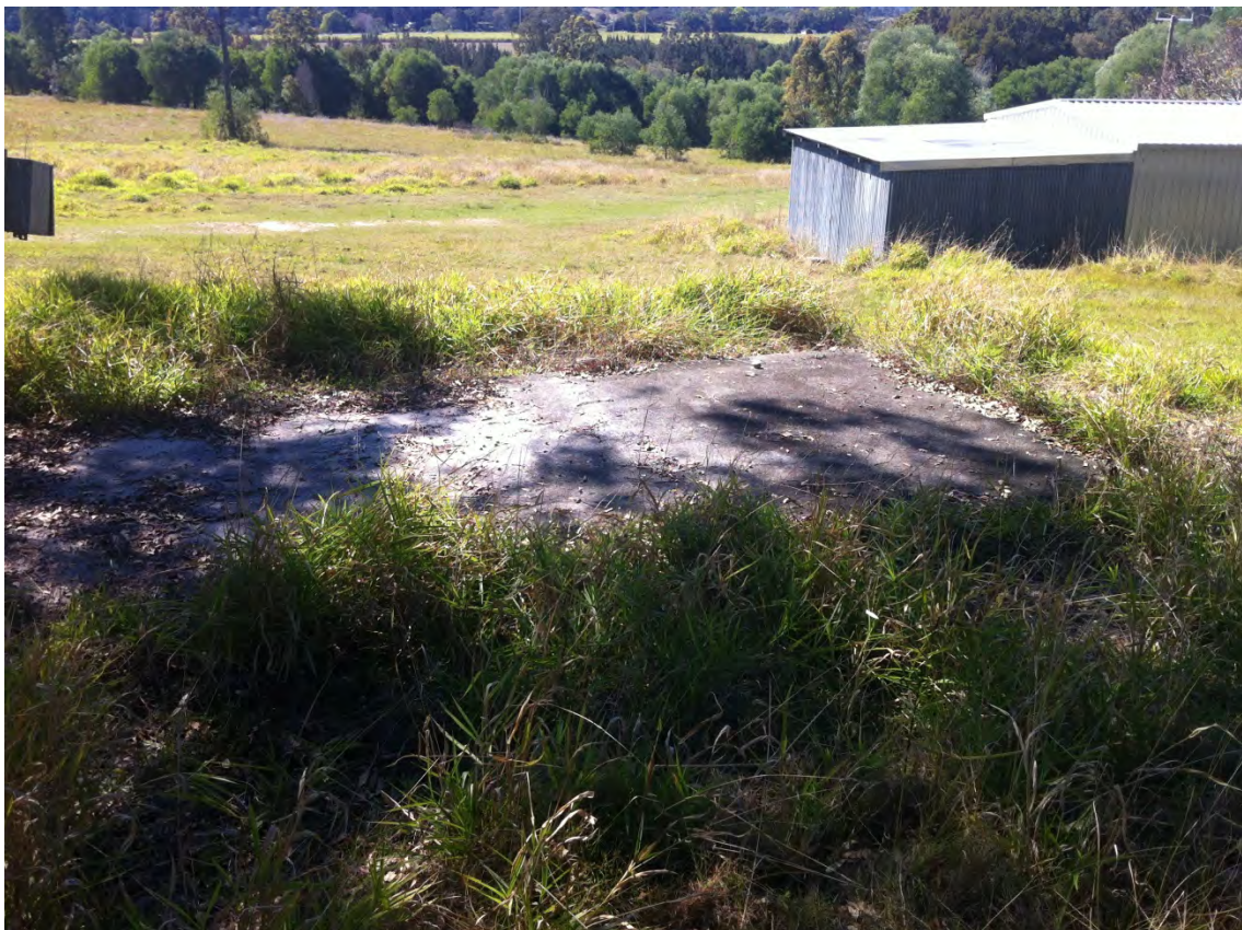
Plate 22 – Concrete slabs to south-west of shed
