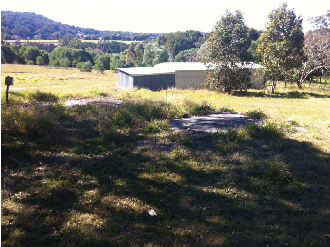
Plate 20 – Concrete slabs to south-west of shed
