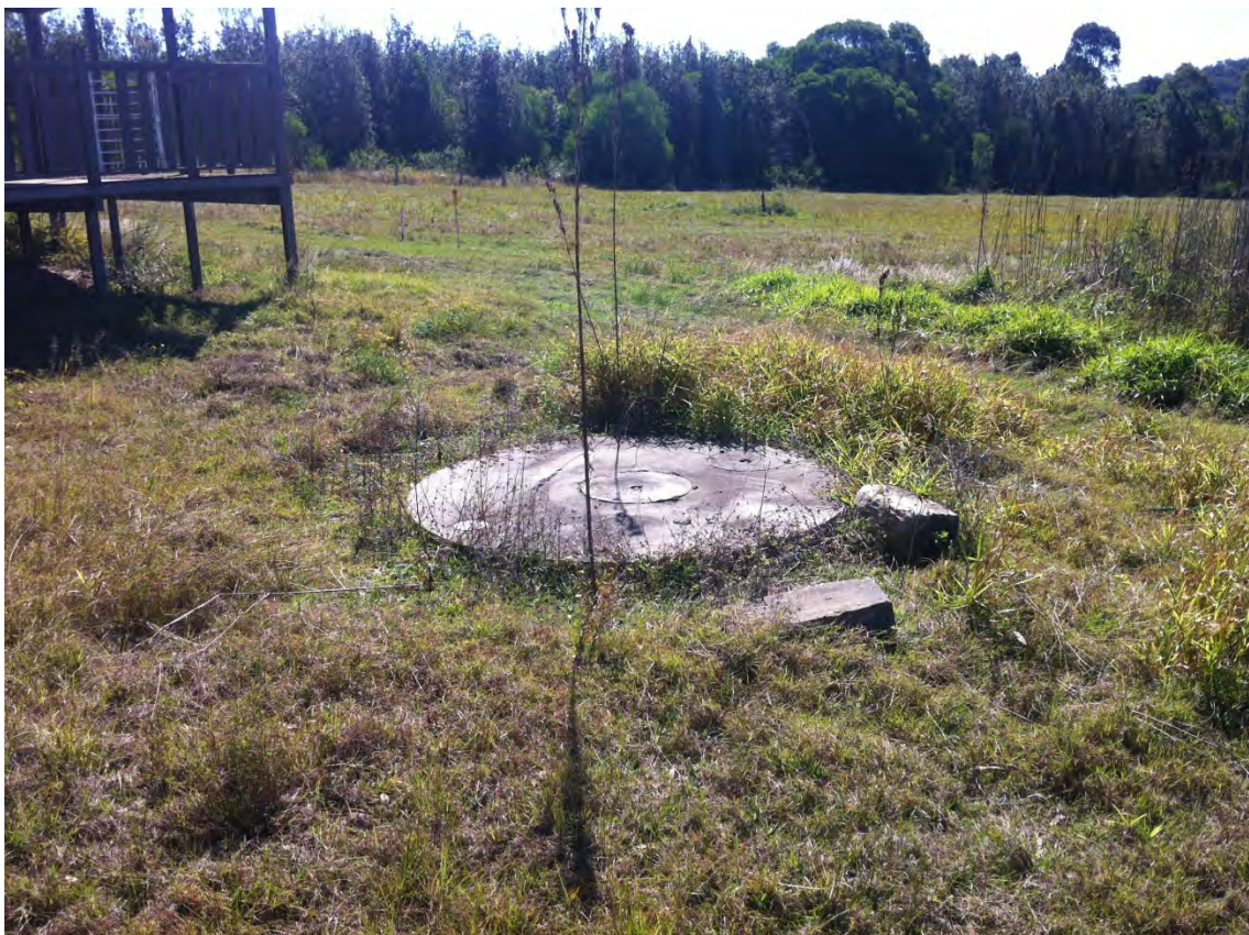
Plate 18 – Circular concrete slab assumed to be septic tank
