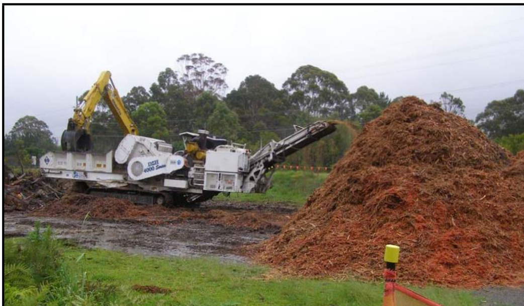
Plate 2: Vegetation mulching activity – mulch should be progressively moved into prepared stockpile areas.
