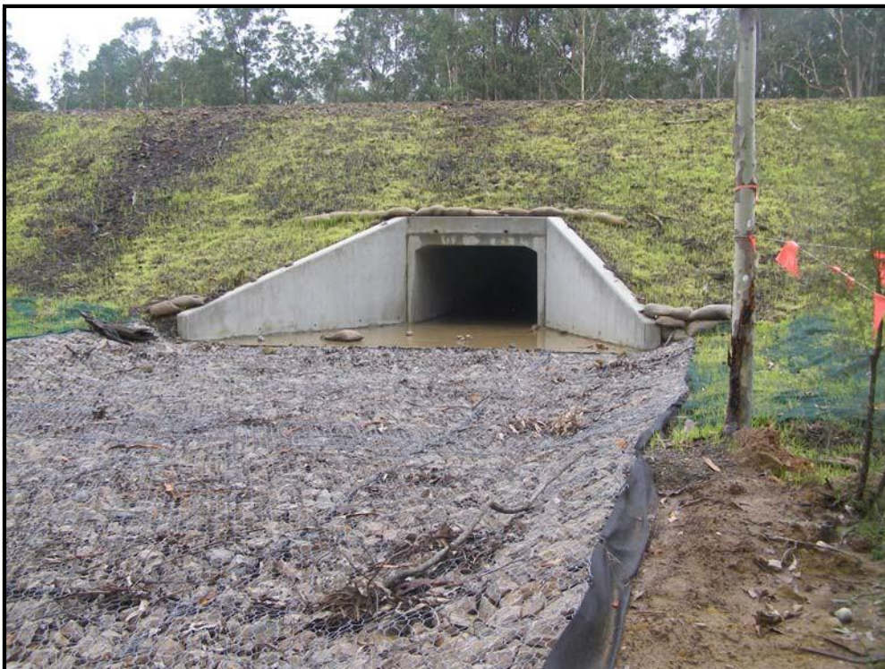
Plate 9: A mulch/topsoil mix used to provide temporary batter stabilisation and to assist cover crop establishment.
