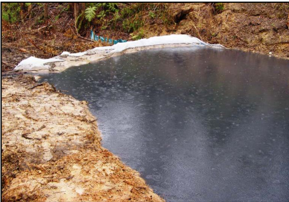
Plate 4: Tannin impact in stormwater at the discharge point from a road construction site. The discharge of impacted water may be obvious to community and other stakeholders.
