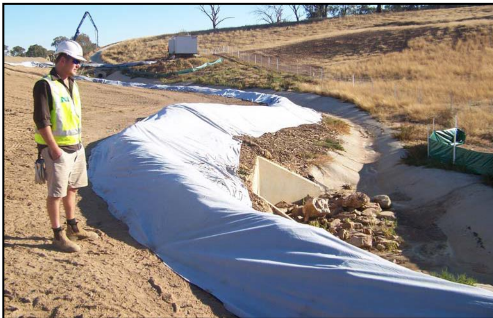
Plate 11: Geofabric wrapped mulch bunds used for sedimentation control
