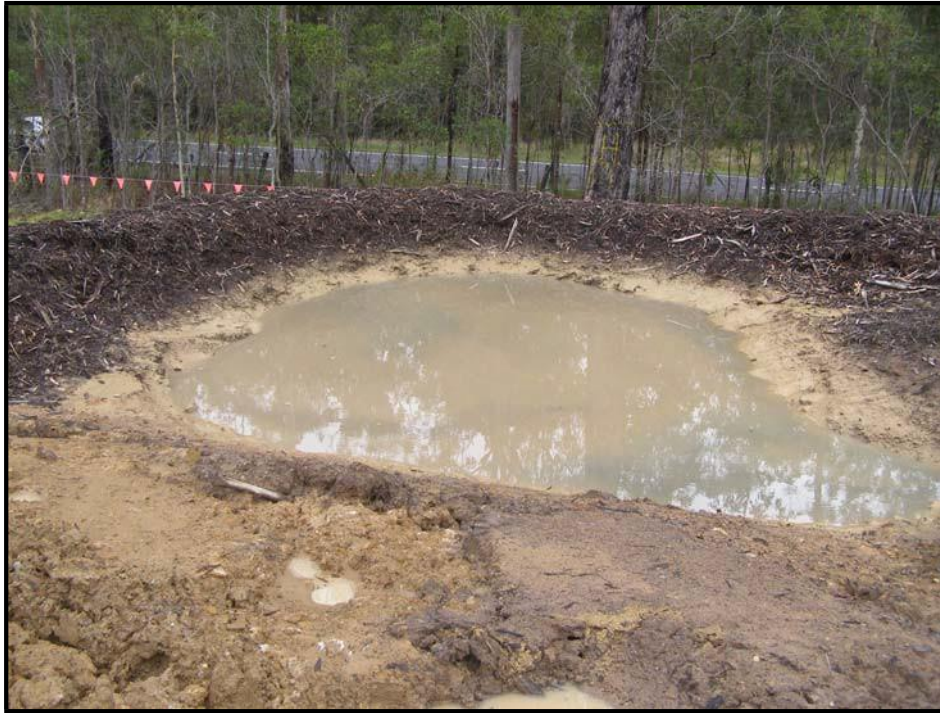
Plate 12: Mulch used as a bund for a temporary sedimentation catch dam. Mulch is effective as it can provide both containment and filtering of site water. Mulch should not be used as a control in areas of concentrated flow where it may be washed away. Any mulch containment control should have a defined and lined outlet that allows discharge from the control without washing mulch away. Note that this control does not have a defined discharge outlet which should be installed to prevent failure of the control in heavy rainfall events.
