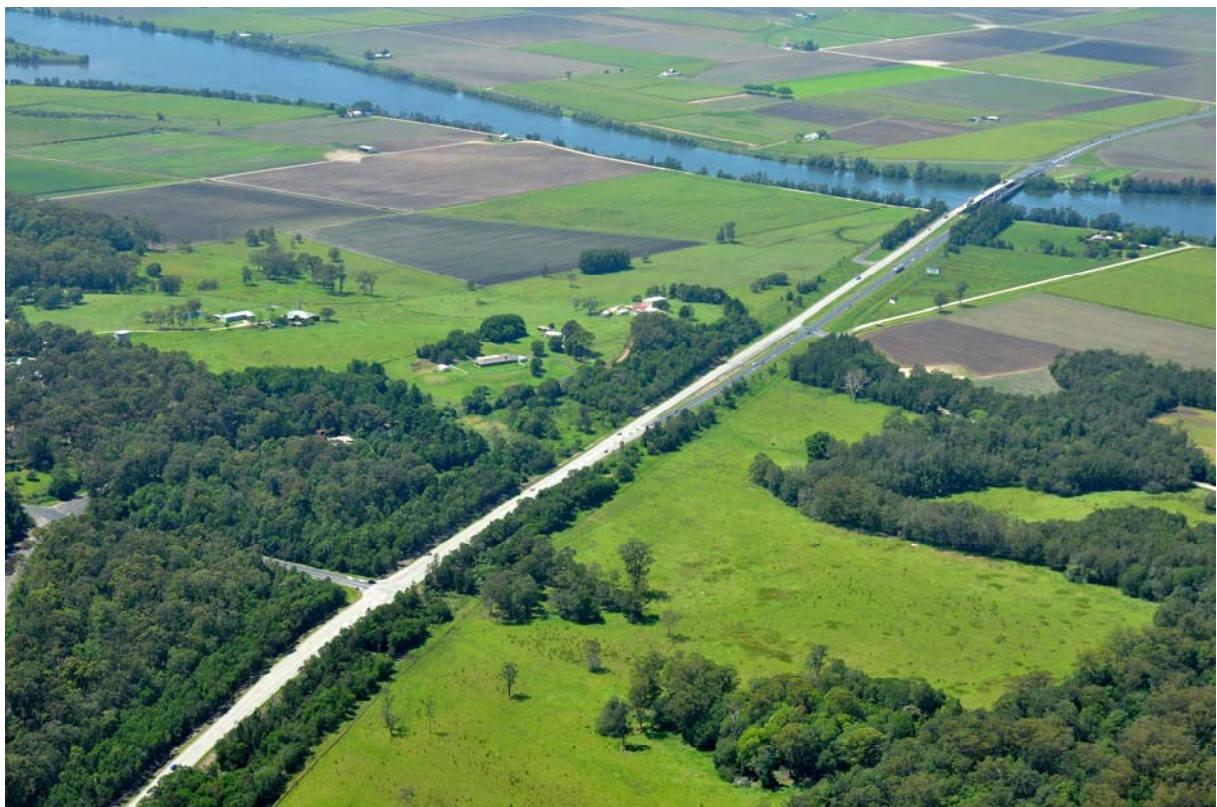
Photo 5: Location of the interchange at Iluka Road, looking towards the Clarence River (North Arm)
