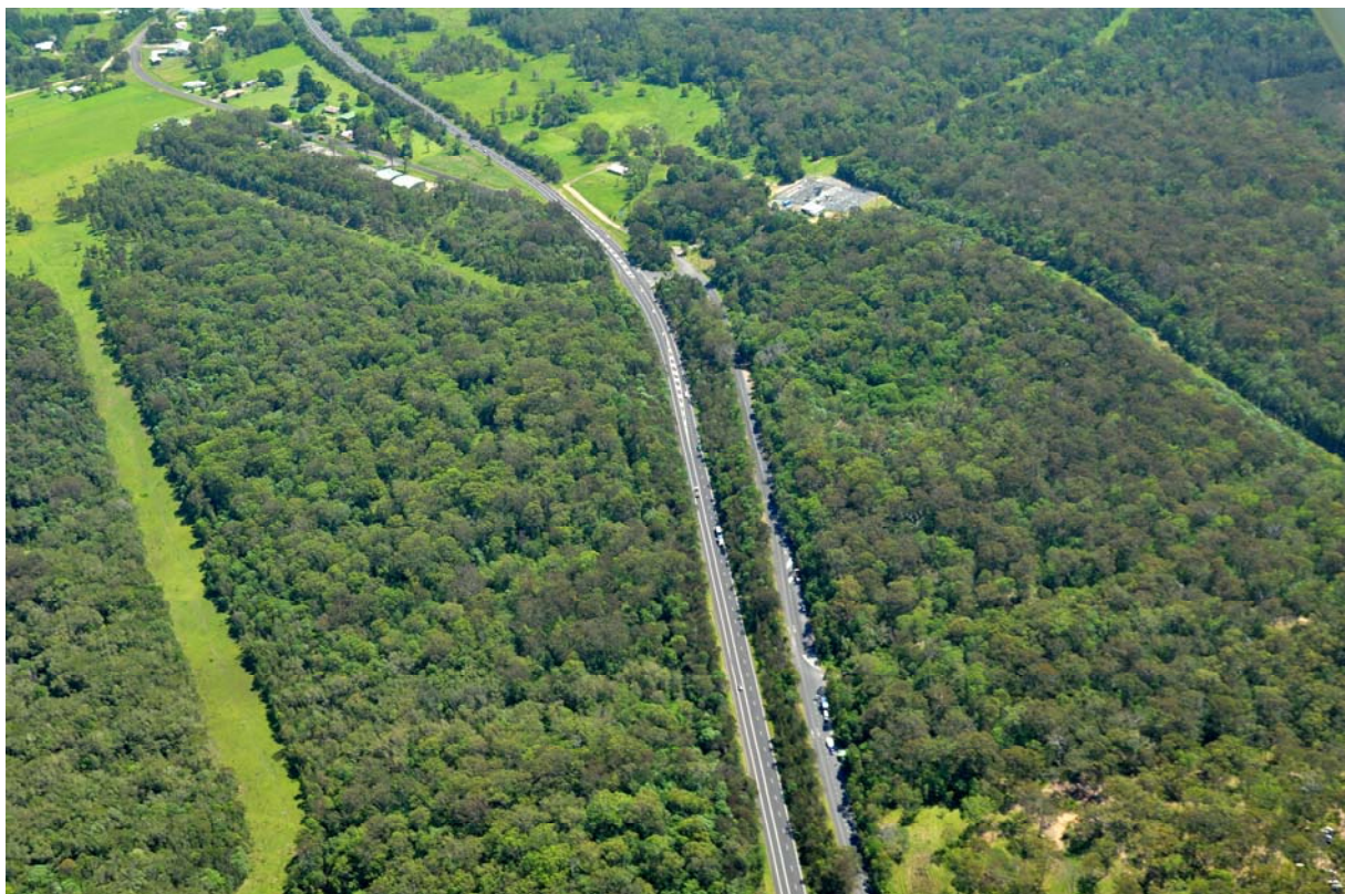
Photo 6: Location of the interchange at Woodburn, looking north.
