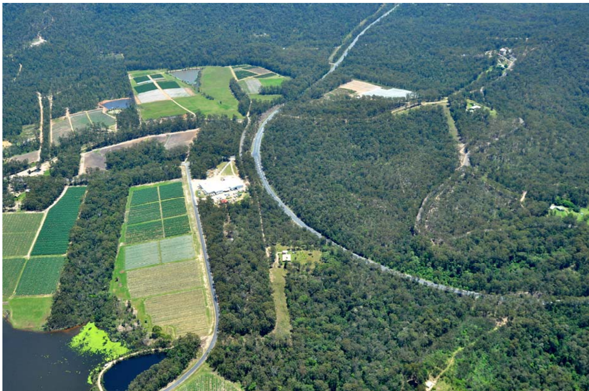
Photo 3: Location of the interchange at Range Road (in foreground)
