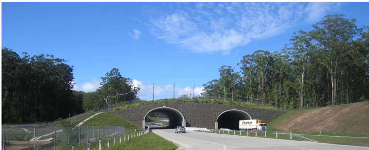
Photo 7: Existing fauna bridge on the Bonville upgrade section of the Pacific Highway
