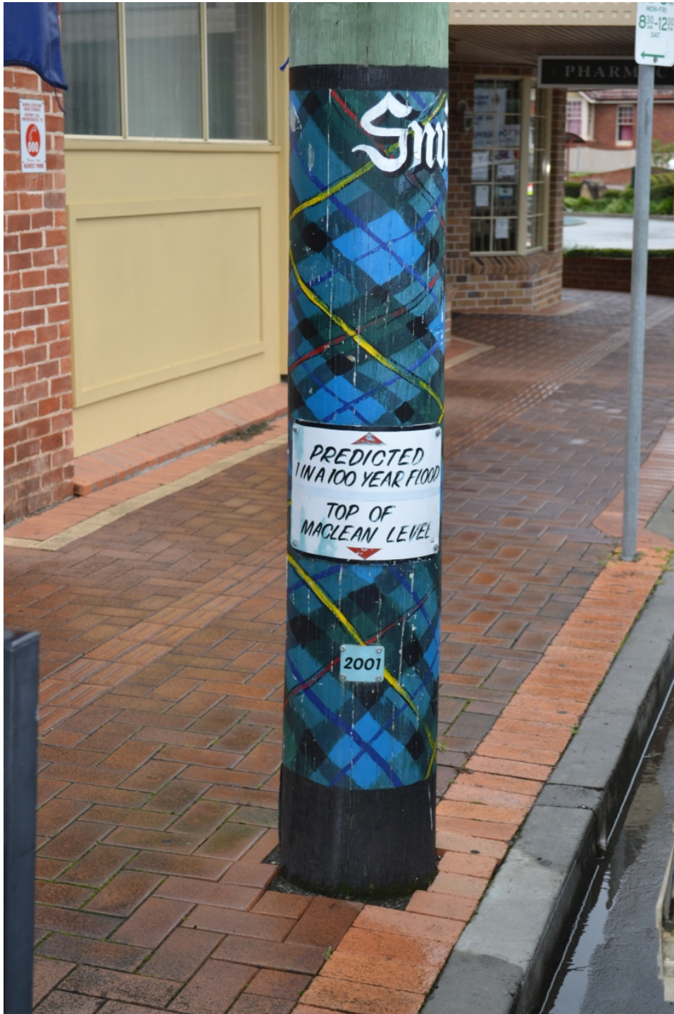
Photo 5: Flood level indicator on main street of Maclean town
