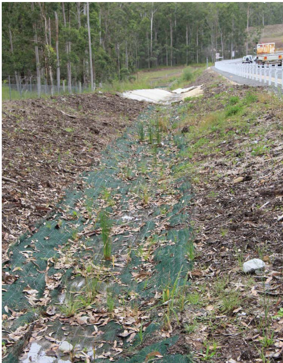
Photo 6: Example of a lined / grassed swale
