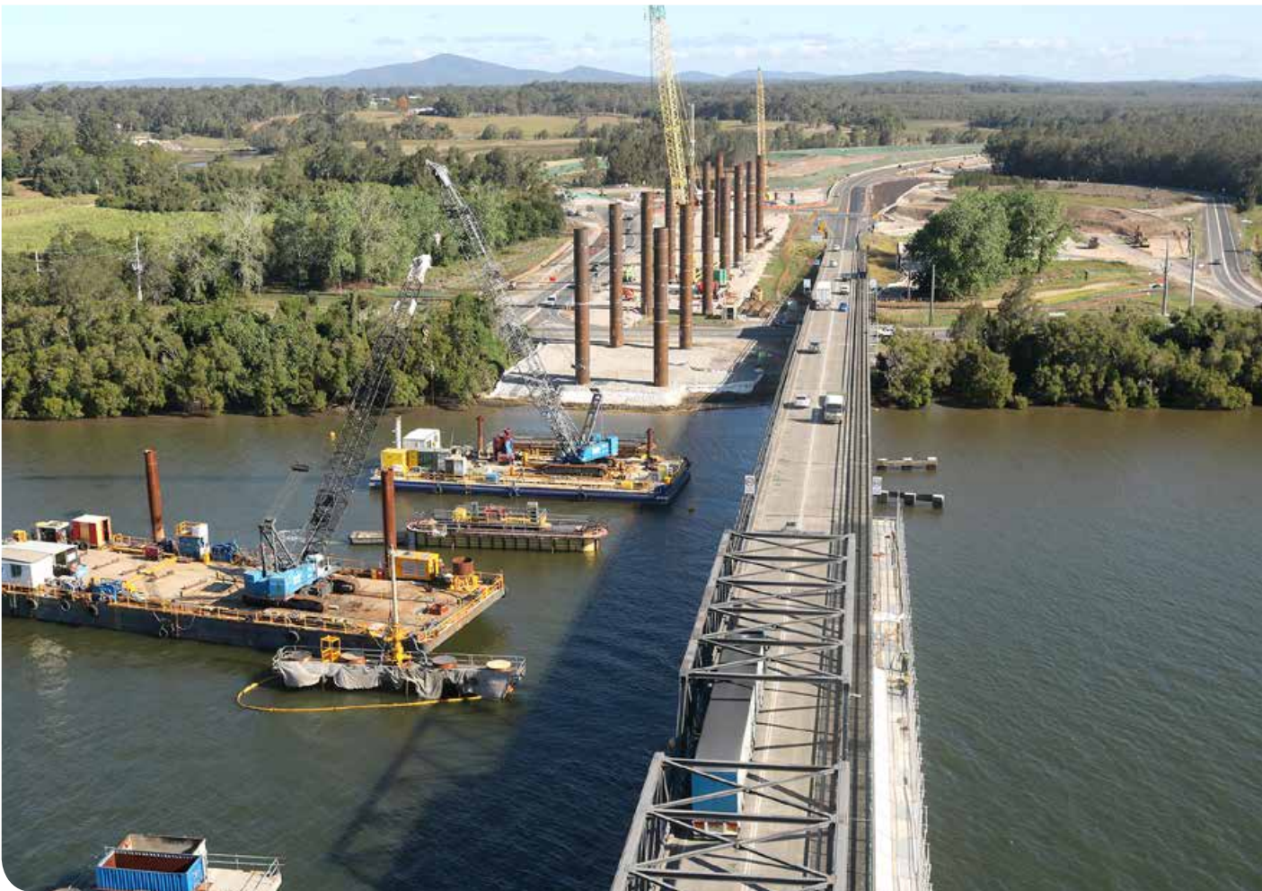
Piling work in the Clarence River and Yamba interchange
