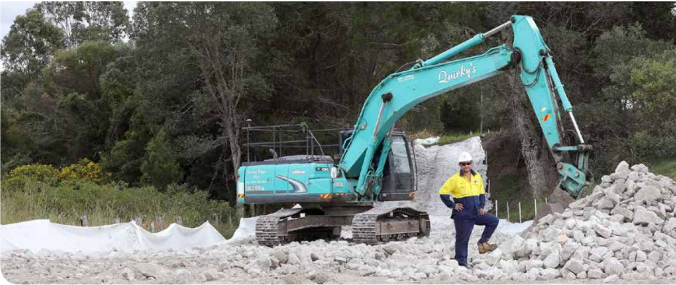
Laying rock for new diversion roads near Iluka Road
