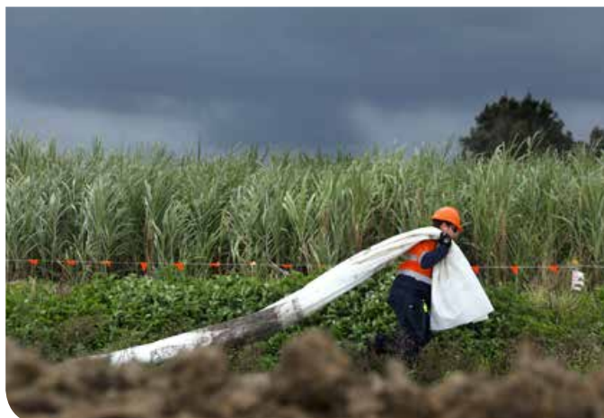
Laying geofabric for new diversion roads on Chatsworth Island
