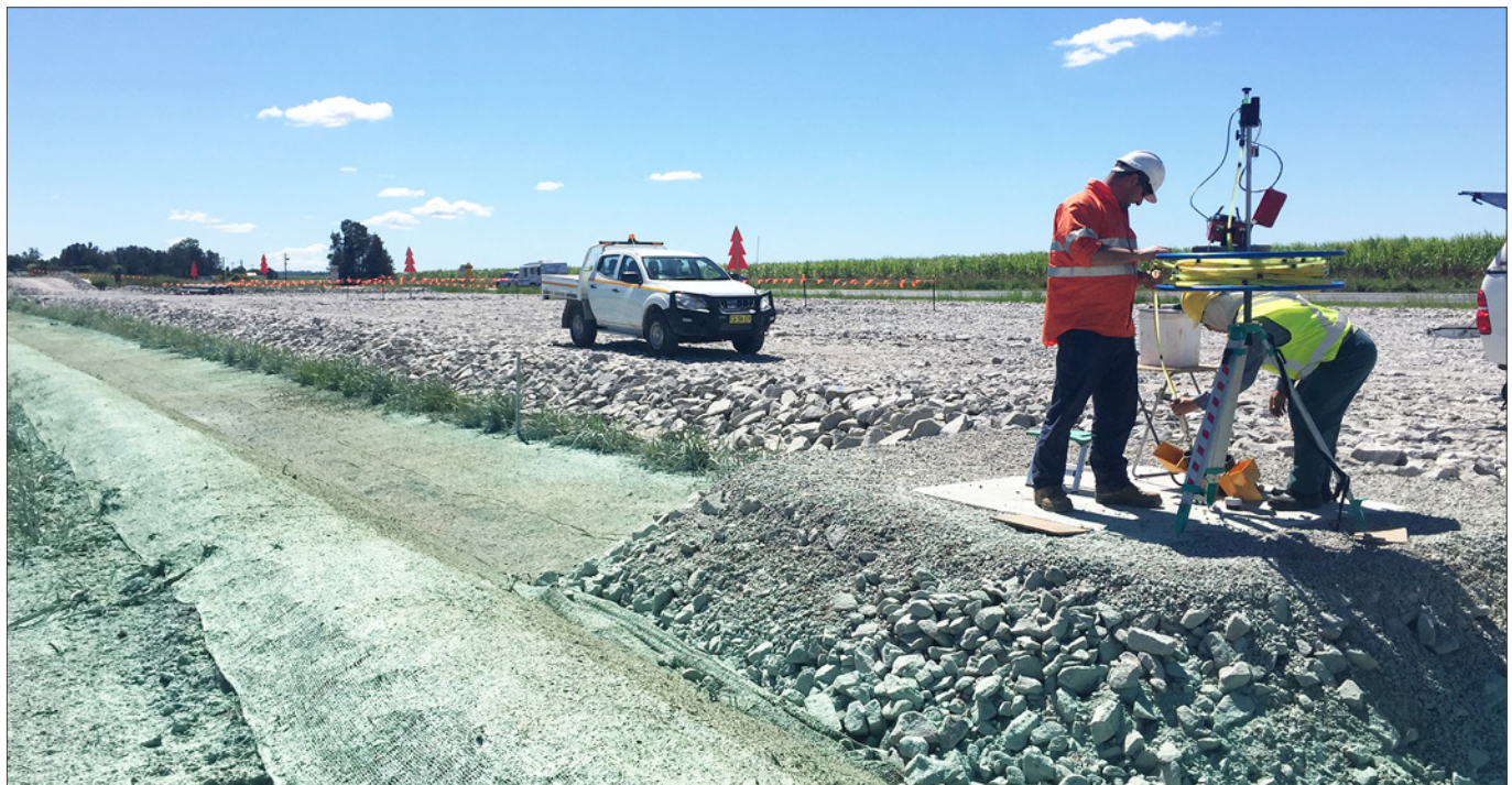
Instrumentation monitoring for soft soil work, showing drainage rock installed
