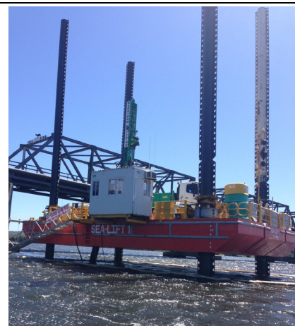
Geotechnical investigations on the river.
