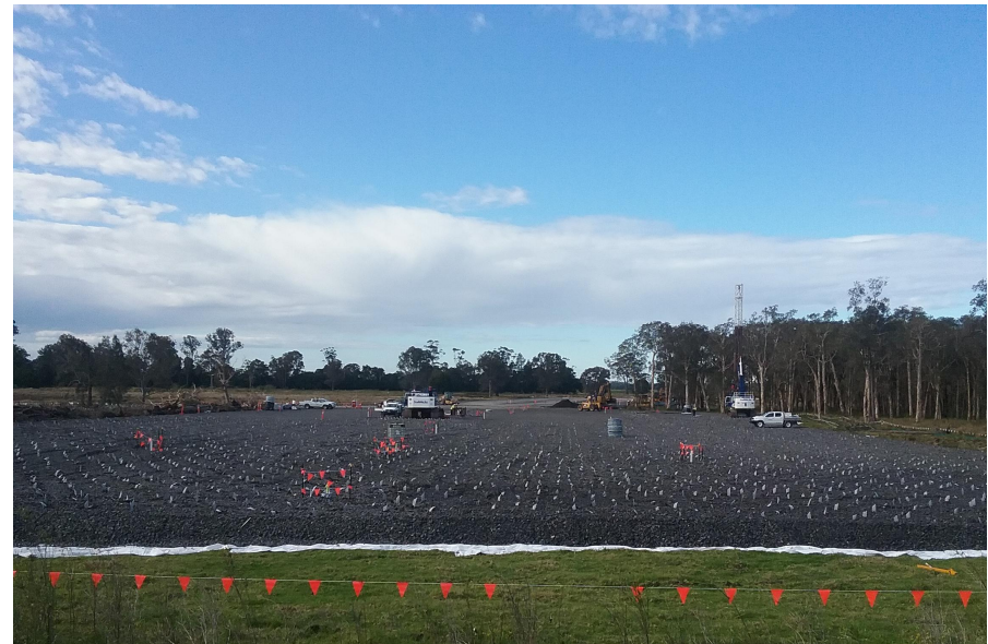
Soft soil work – foundation rock being placed
