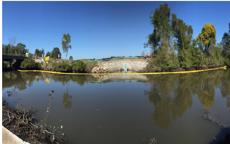
Environmental controls at Serpentine Channel
