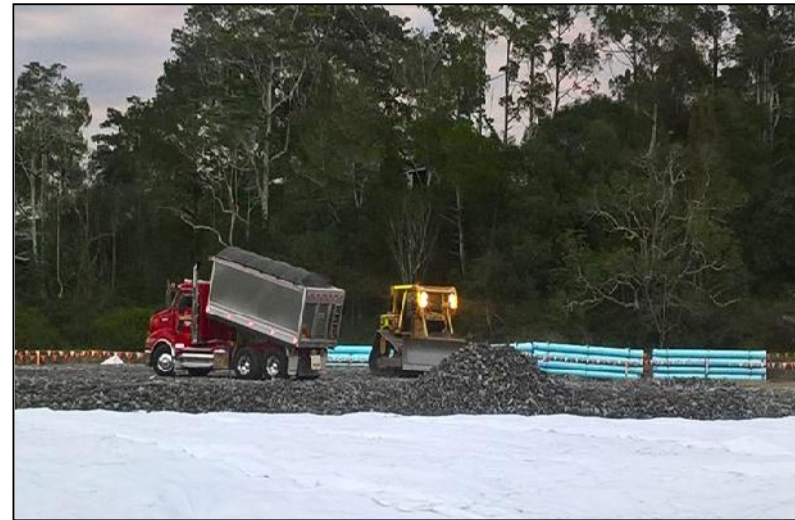
Soft soil work – foundation rock being placed at Ferry Park, Maclean
