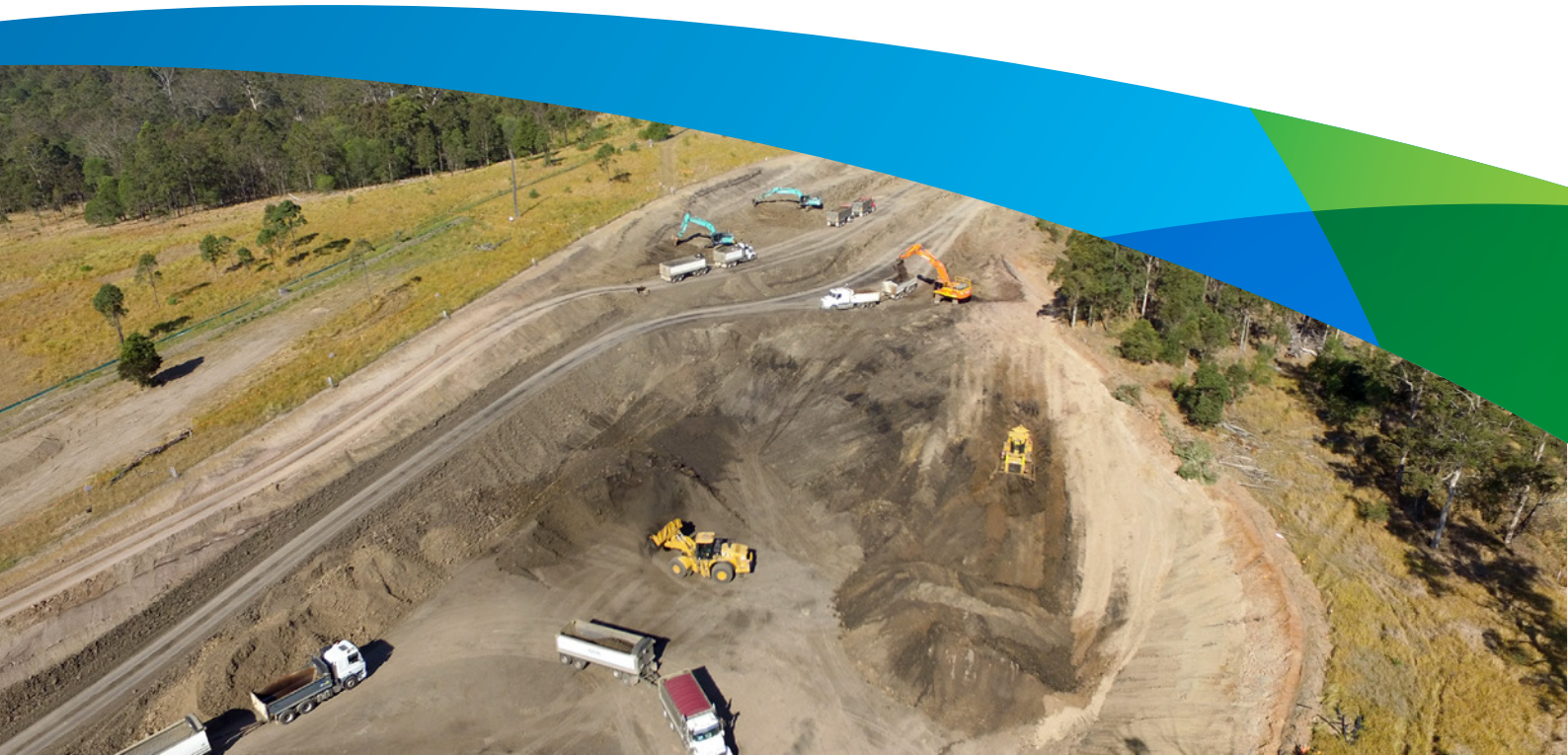
Aerial view of earthwork in progress for Wave 1 soft soil work
