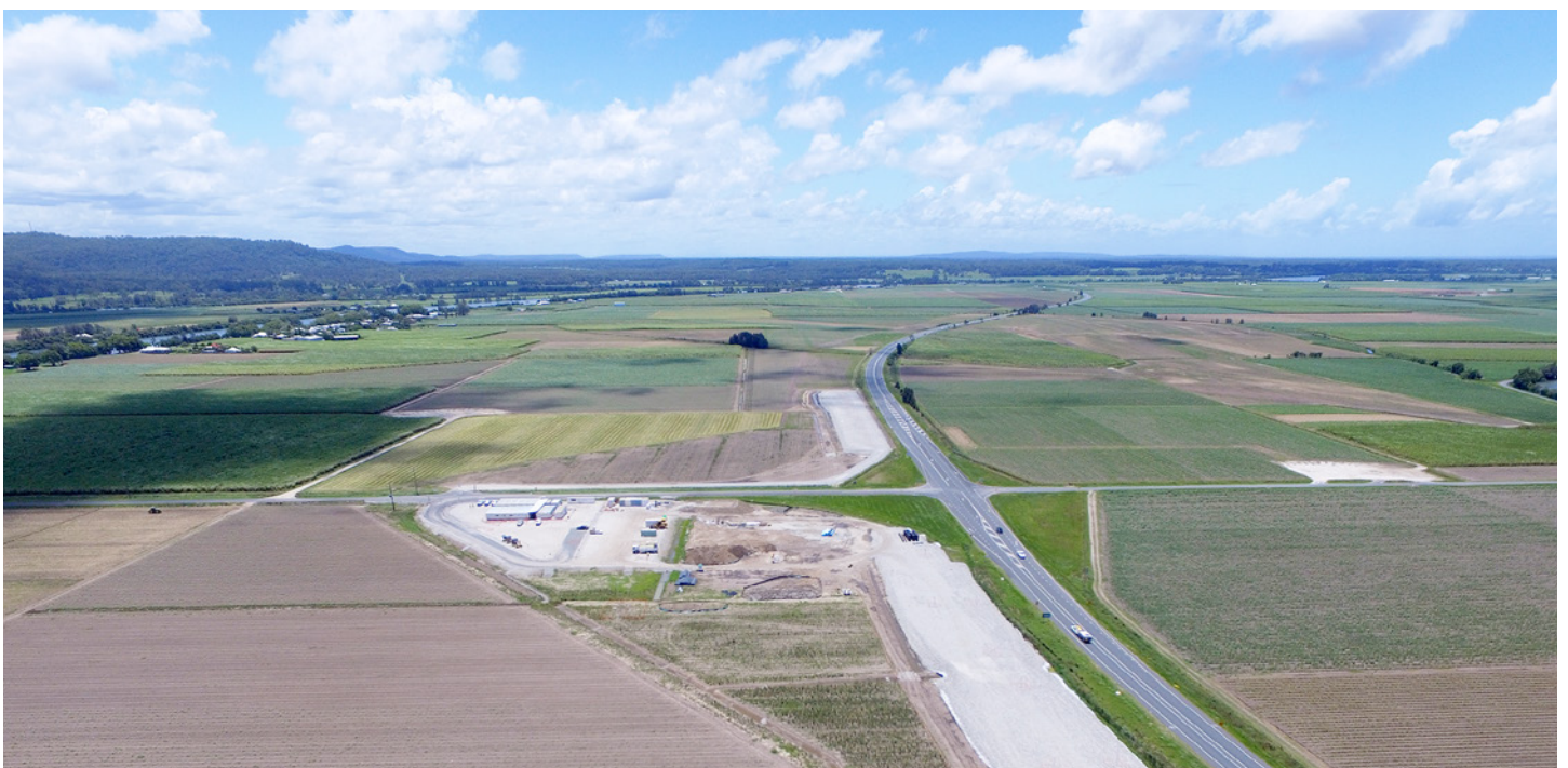
Chatsworth Island: View facing north to Chatsworth Road
