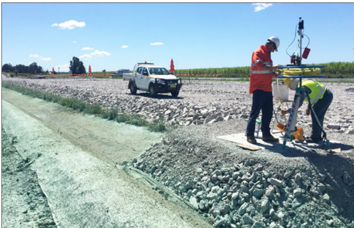
Monitoring for soft soil work at Farlows Flat in March 2016
