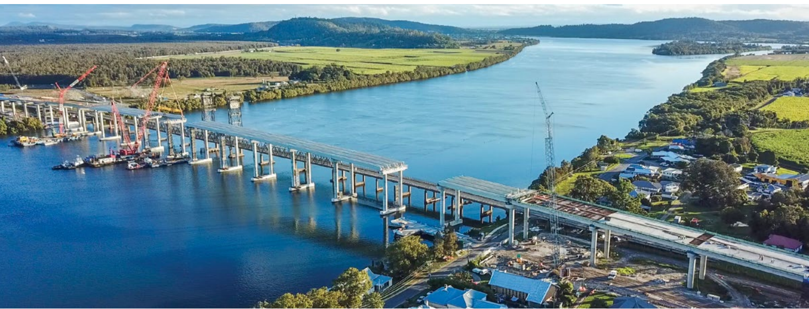
New bridge over the Clarence River at Harwood
