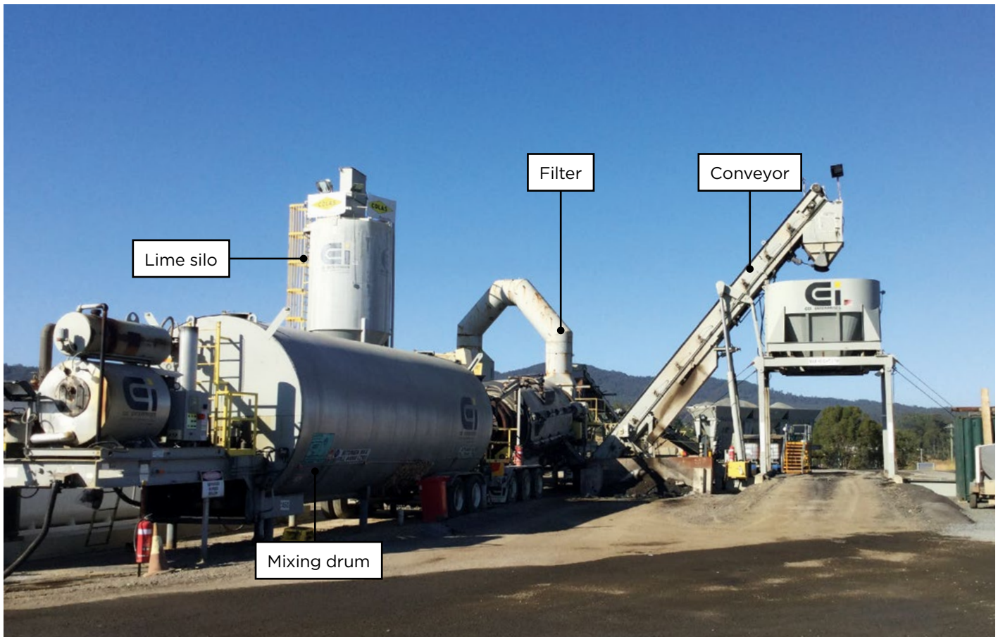
Temporary asphalt batch plant for the Warrell Creek to Nambucca Heads section of the Pacific Highway upgrade
