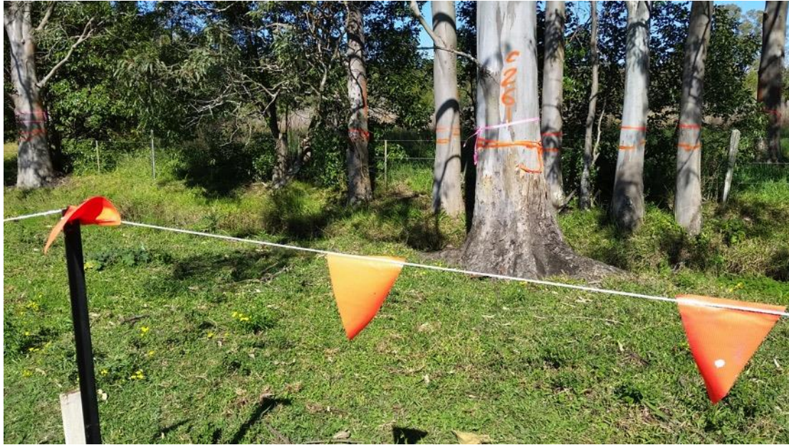
Plate 1: Delineation of the Limit of Clearing (LoC) boundary at Wardell Road. A collared tree is shown in the background.
