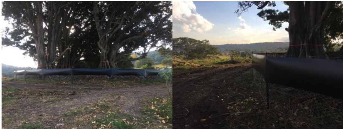
Plate 3: Combined chicken wire and HDPE fence installed around two clusters of large fig trees that could not be collared.
