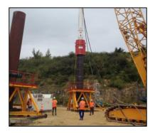
**Bored piling** involves boring a circular hole in the ground, installing steel reinforcement and filling the bore hole with concrete to form a pile.
