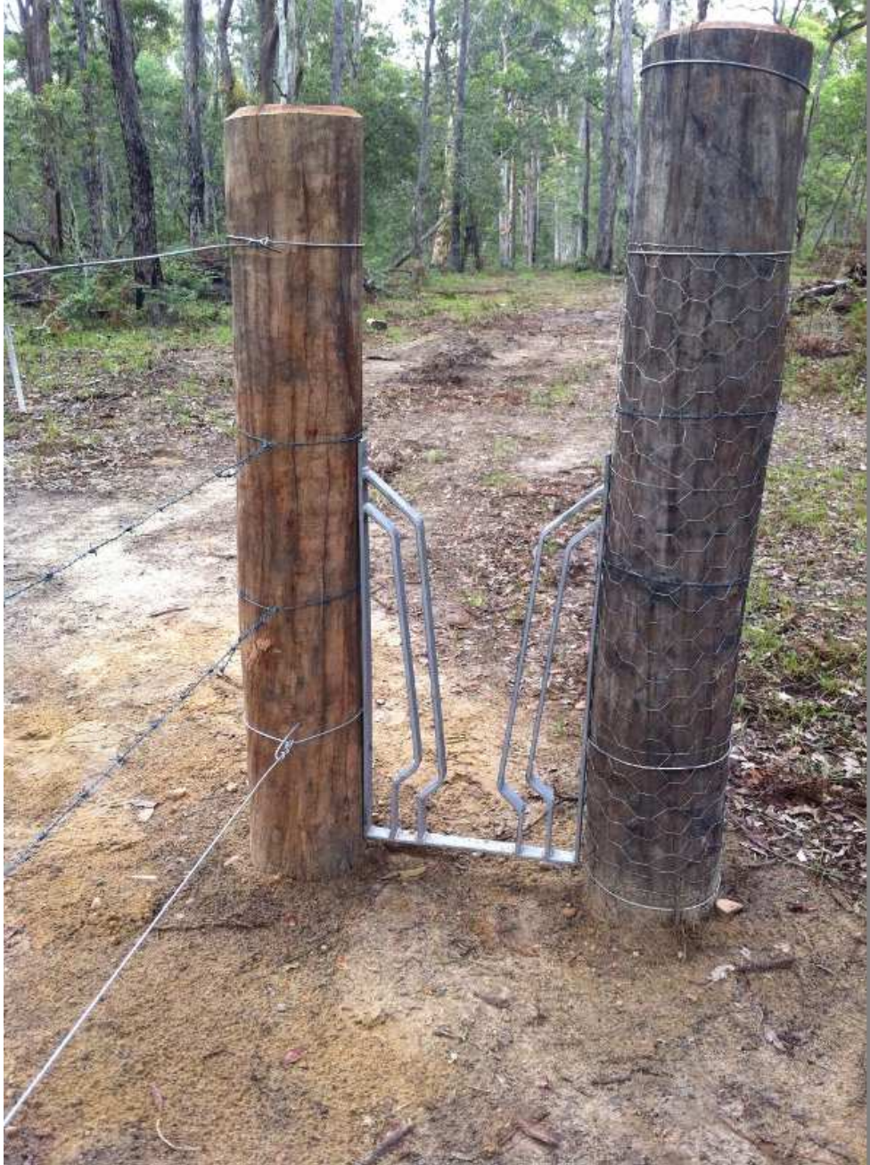
Figure 3-3 Temporary emu squeeze style fence
