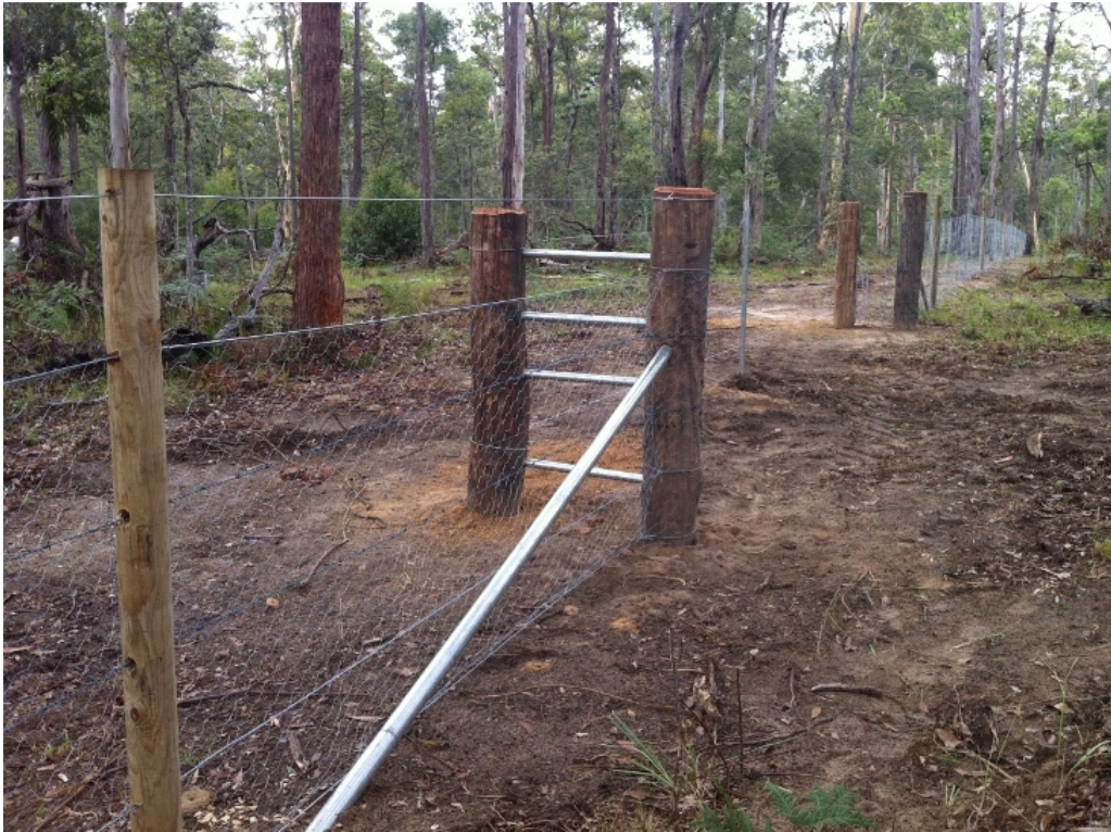
Figure 3-2 Temporary emu fence and bollard gate
