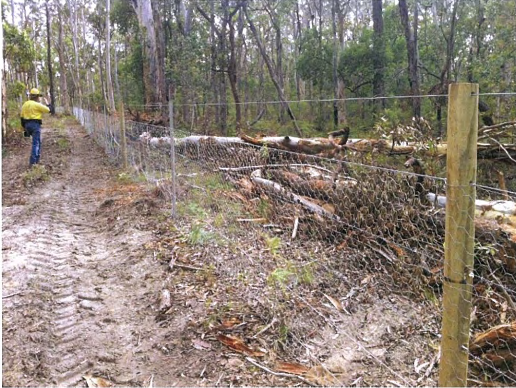
Figure 3-1 Temporary emu fencing
