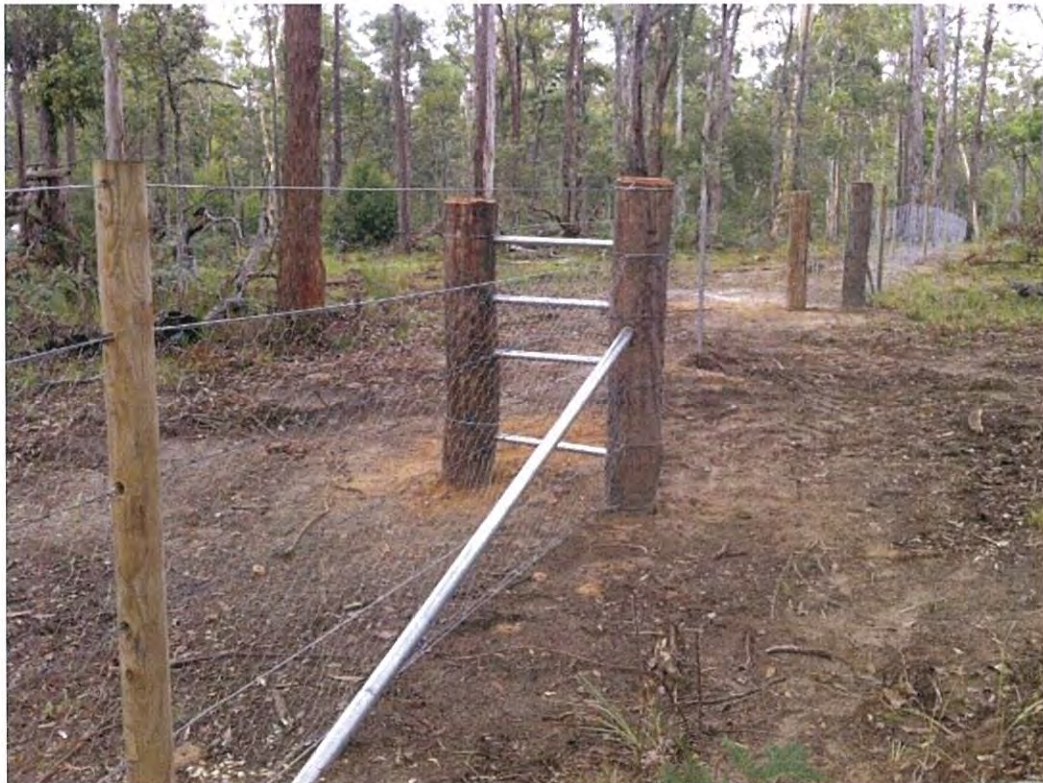
Figure 3-2 Temporary emu fence and bollard gate
