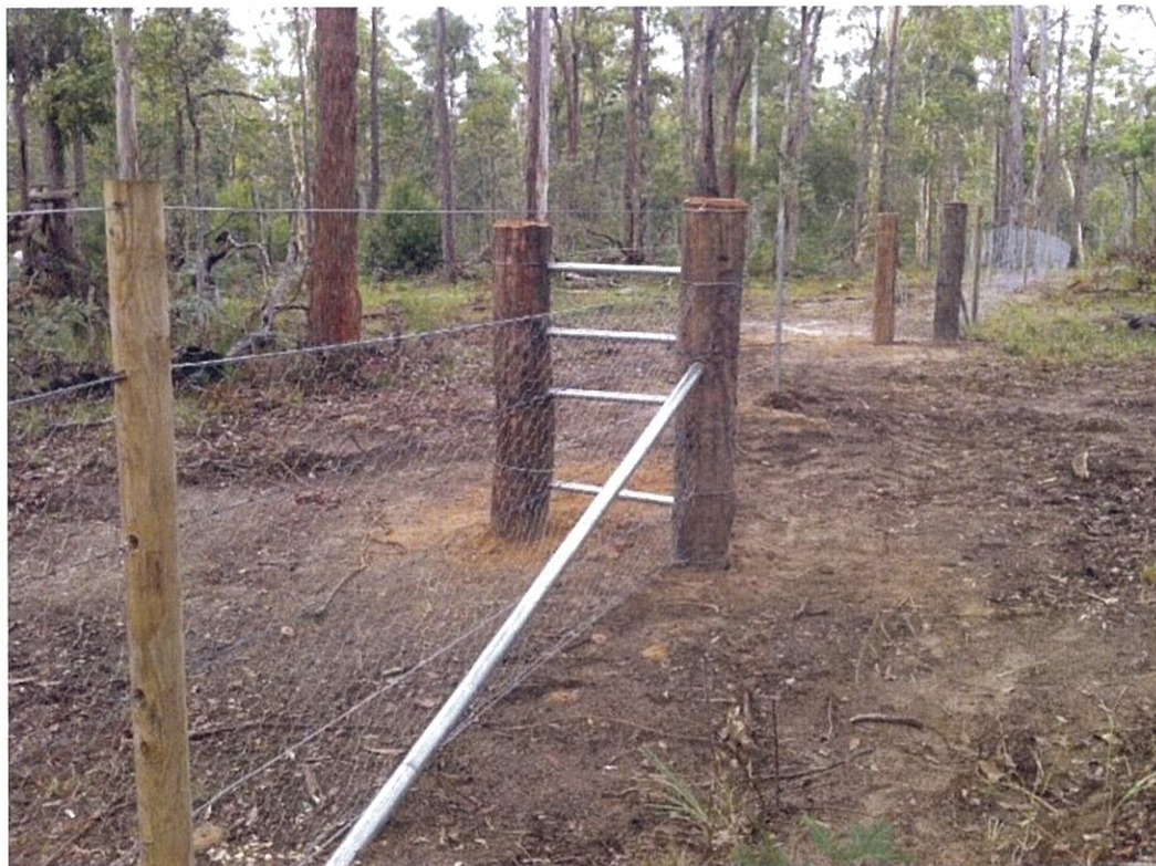
Figure 3-2 Temporary emu fence and bollard gate
