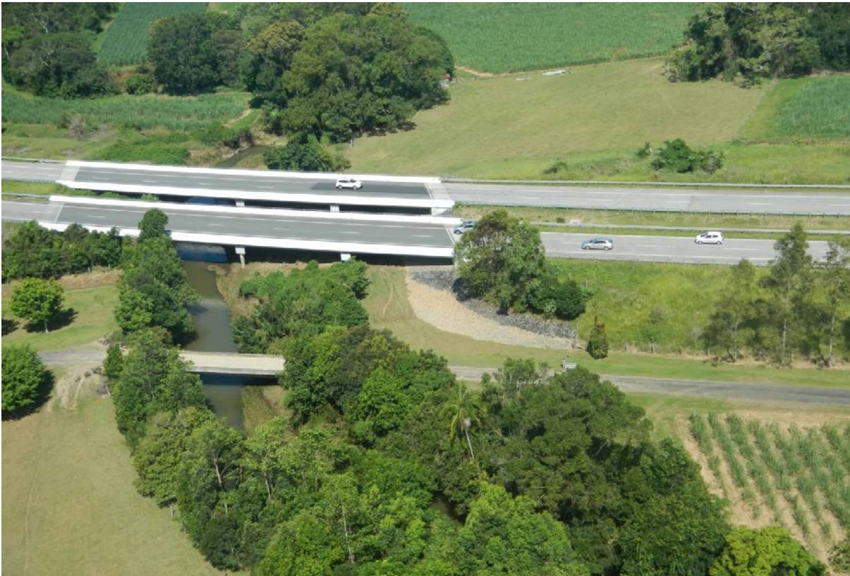
Plate C -6 Burringbar Creek (1 February 2013, 2.24pm), showing no evidence of debris blockage.
