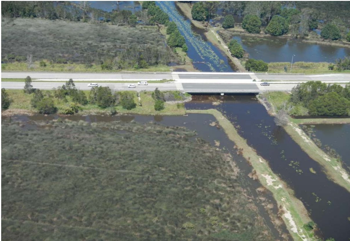
Plate C -3 Clothiers Creek (1 February 2013, 2.16pm), showing no evidence of debris blockage.
