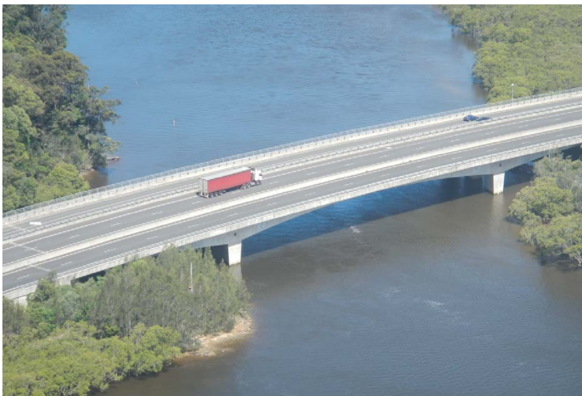
Plate C -8 Brunswick River (1 February 2013, 2.29pm), showing no evidence of debris blockage.
