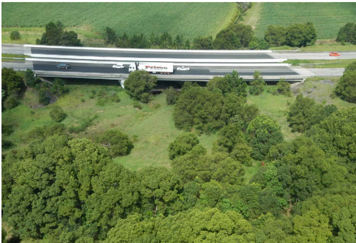
Plate C -7 Crabbes Creek (1 February 2013, 2.25pm), showing no evidence of debris blockage.
