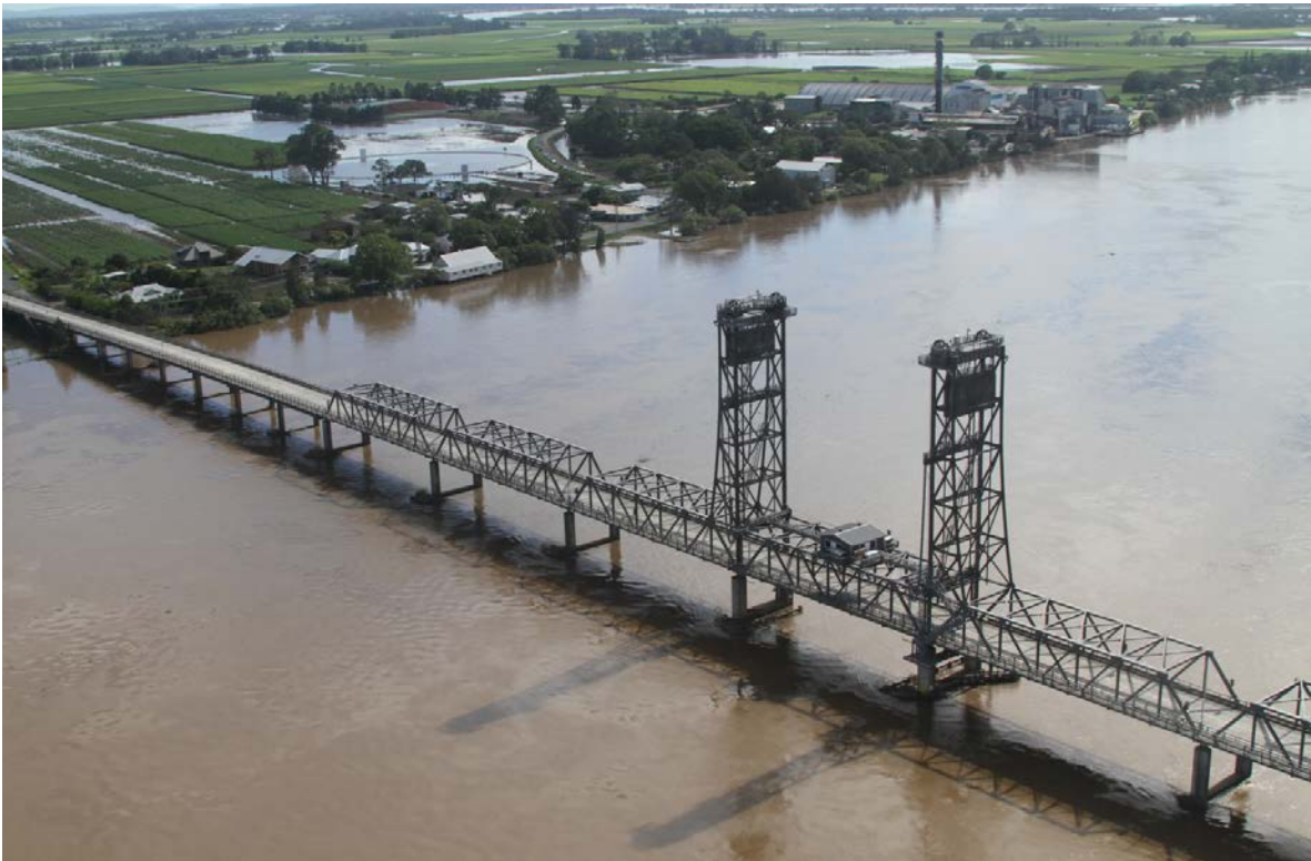
Plate C -13 Clarence River Main Arm (Harwood Bridge) (31 January 2013, 9am-10am), showing moderate evidence of debris blockage around bridge piers.
