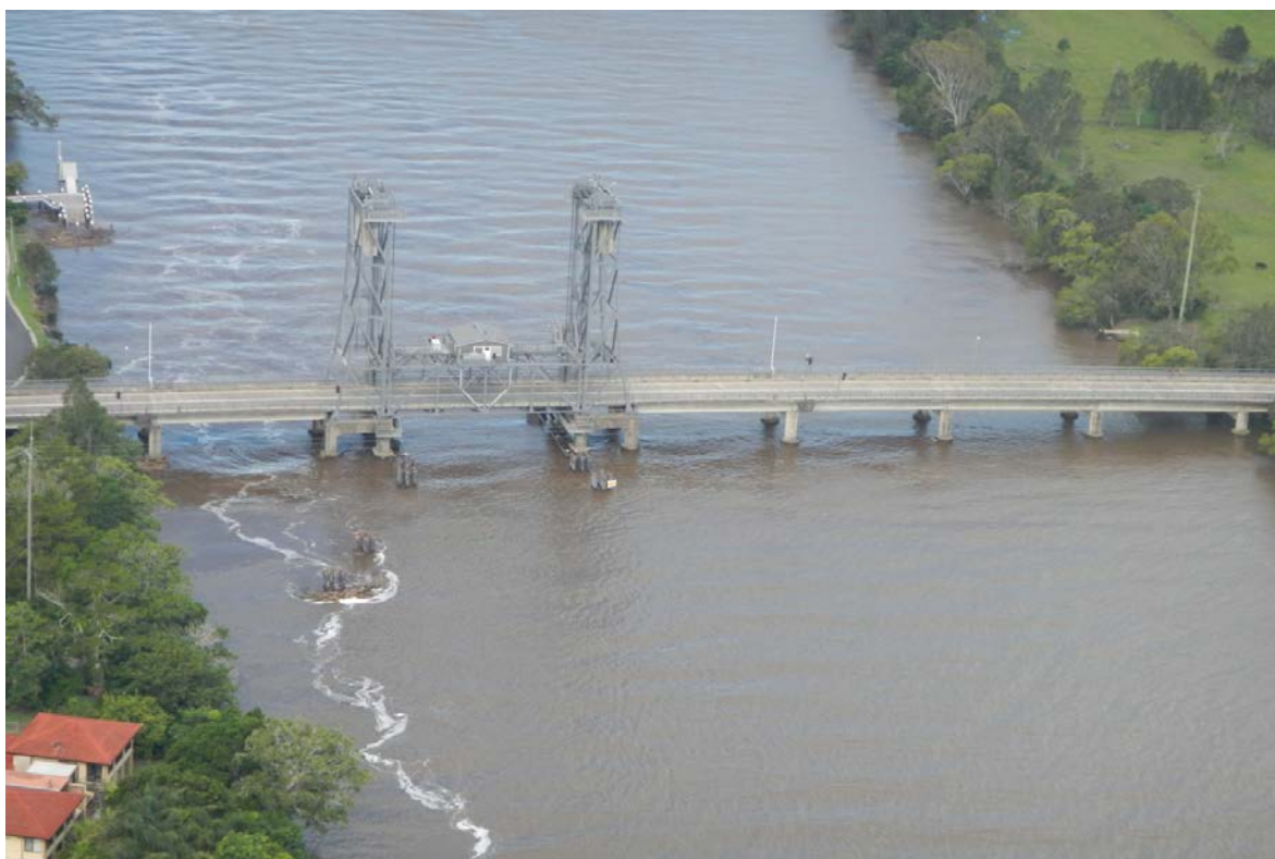
Plate C -12 Richmond River (Wardell Bridge) (1 February 2013, 3.10pm), showing no evidence of debris blockage.
